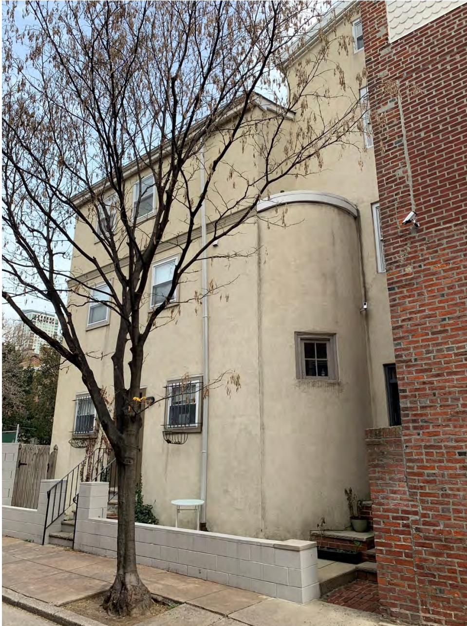
Figure 7: The curved corners of the original two-story rear ells of 919 and 921 Lombard Street are shown in historic maps, and remain visible following a third-floor addition constructed in 2000. December 2021.
