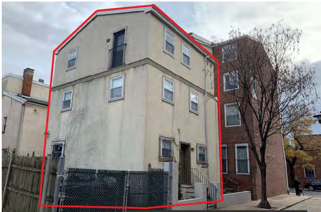
Figure C: North and west elevations of rear of 919-21 Lombard St. Area of new construction in 2000 outlined in red. Both rear ells were constructed in 2000. Foundation remained in place.
