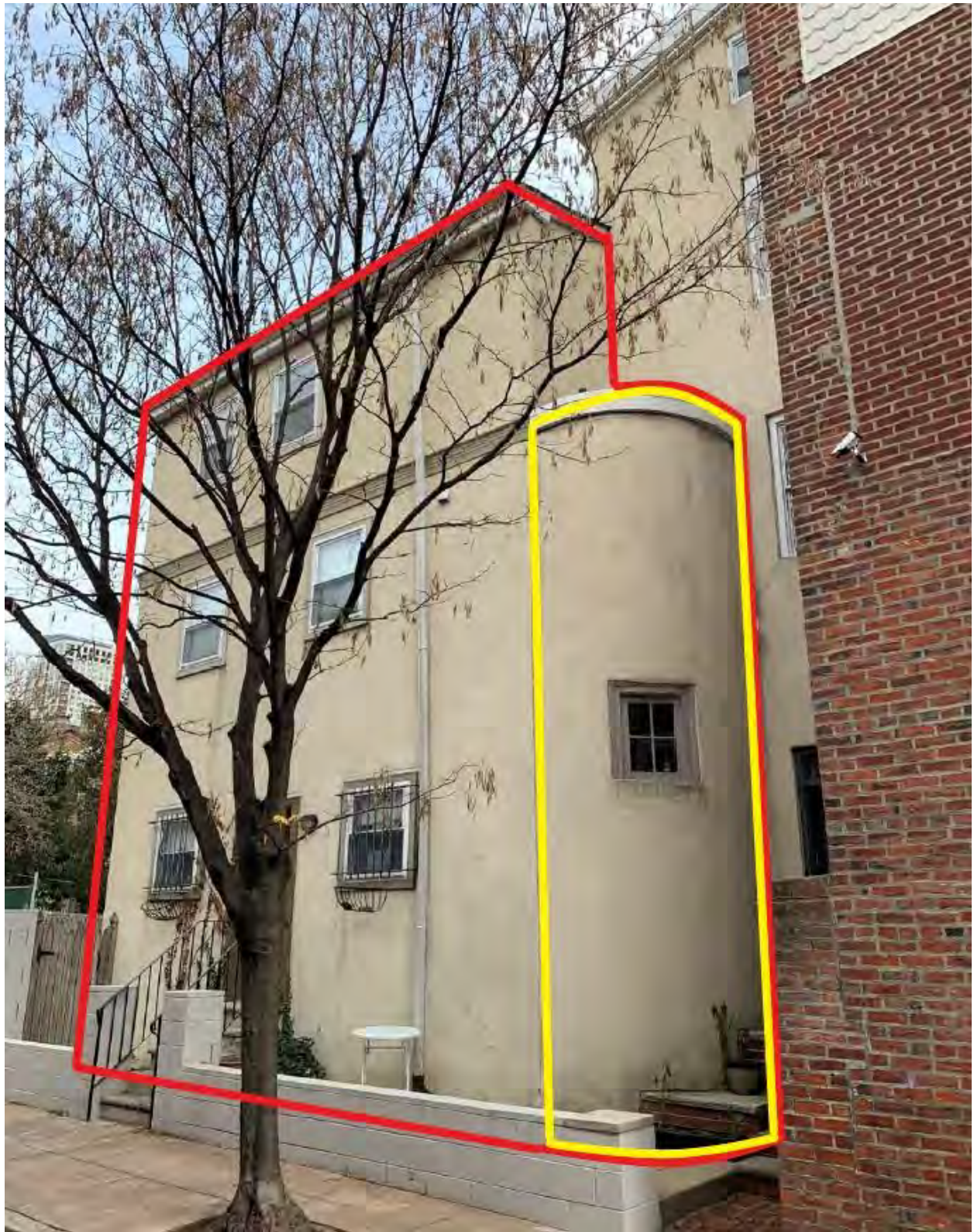
Figure D: Area of 2000 construction indicated in red. The new construction occurred on top of existing foundation. The curved wall areas on west and east elevations (outlined in yellow) were partially reconstructed and are a mix of older brick and new concrete block.
