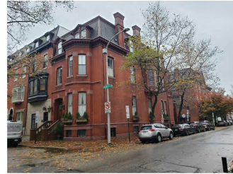
EXISTING PHOTO (11/30/2020) FROM NORTH EAST CORNER, LOOKING SOUTH WEST
