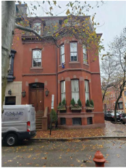
EXISTING PHOTO (11/30/2020) NORTH ELEVATION
