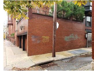
EXISTING PHOTO (11/30/2020) SOUTH ELEVATION
