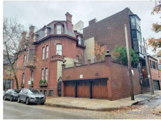
EXISTING PHOTO (11/30/2020) FROM SOUTH WEST CORNER, LOOKING NORTH WEST
