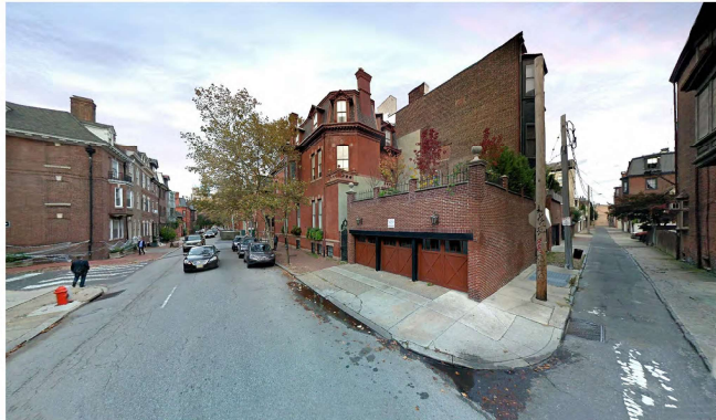
EXISTING STREET VIEW OF GARAGE FROM SW CORNER
