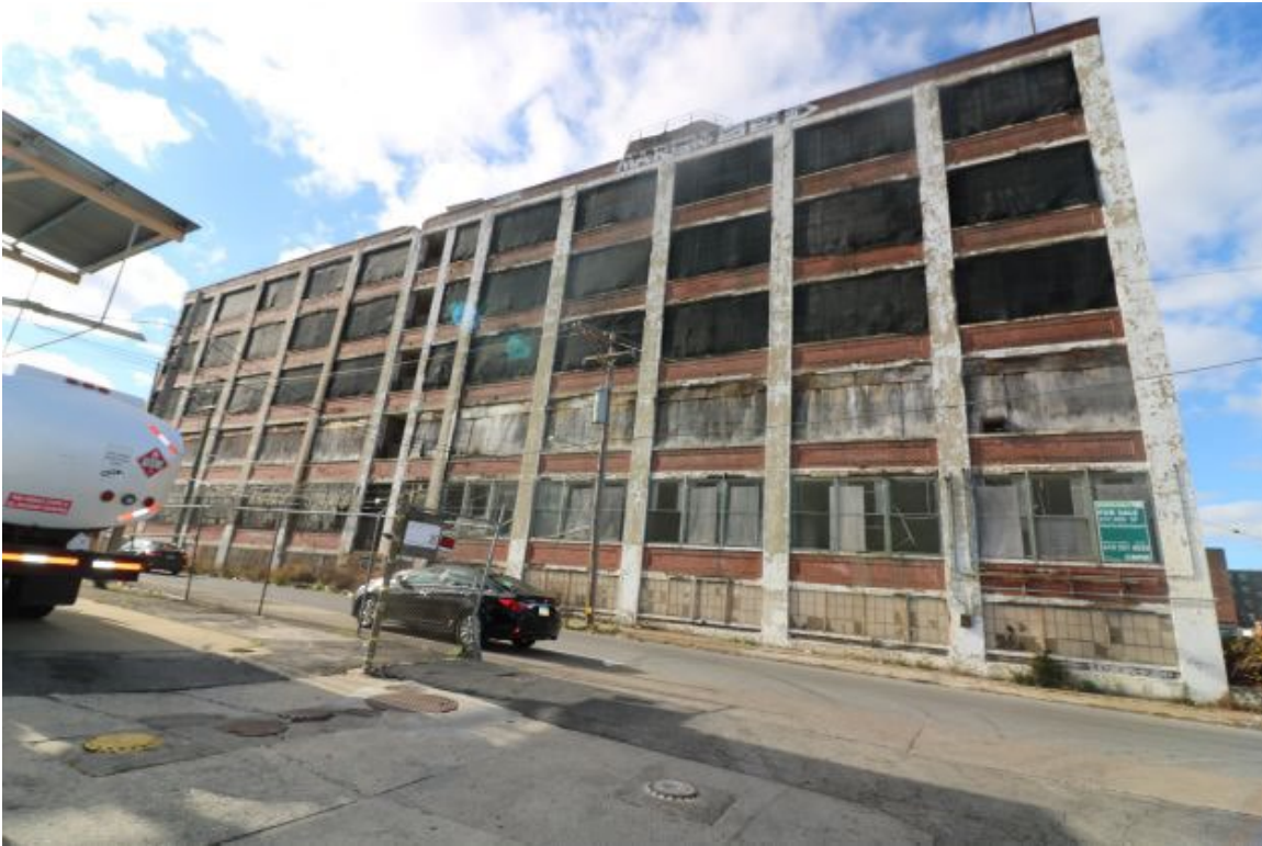
Figure 7: Plant, East (N. 21st Street) Elevation, view looking west.
