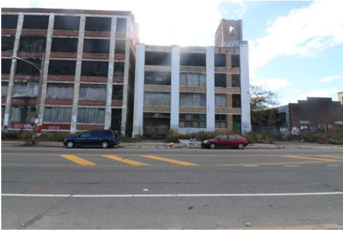
Figure 12: Main Office Building, North (W. Allegheny Ave.) Elevation, view looking south.
