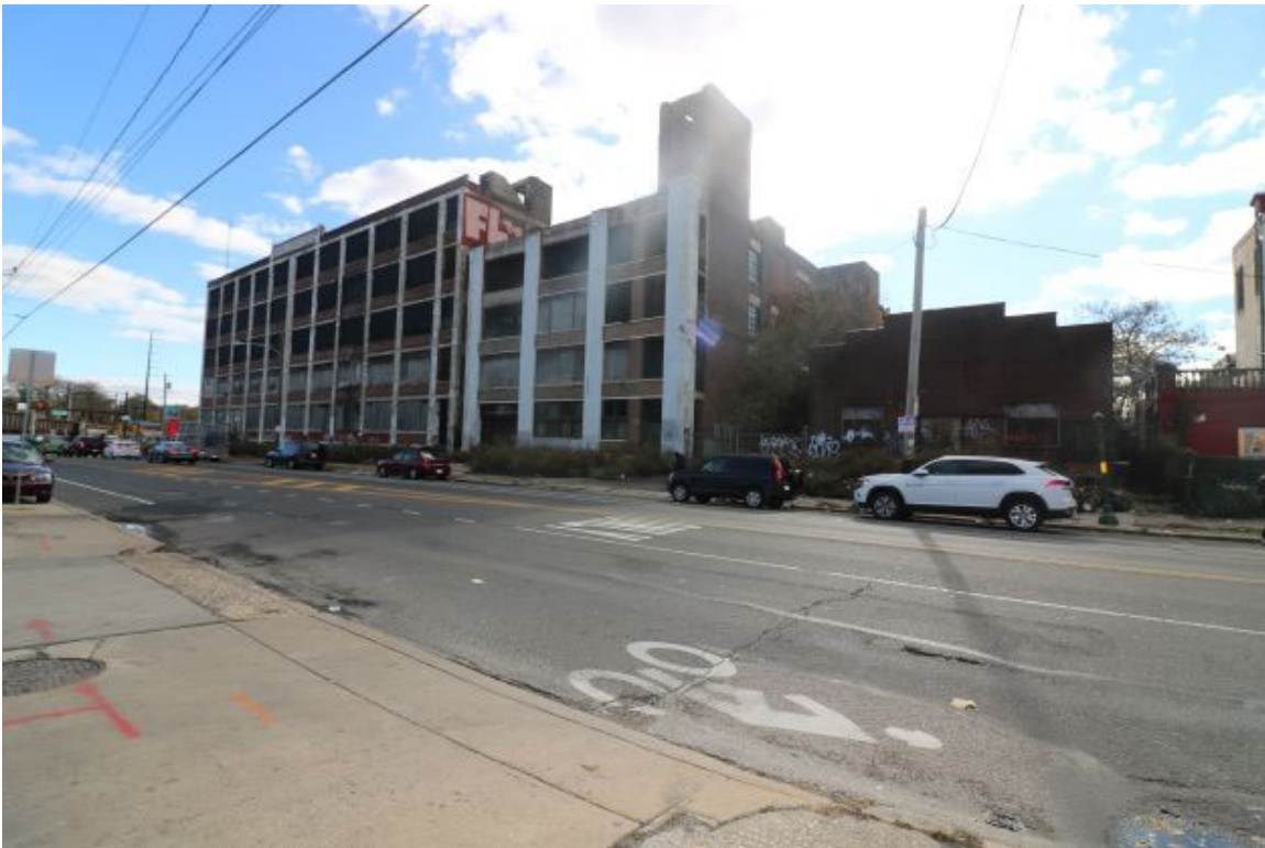
Figure 4: Steel Heddle Manufacturing Company Complex, view looking southeast.
