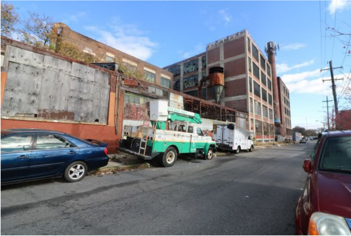
Figure 14: Lumber Storage-Garage Building, South (W. Lippincott St.) Elevation, view looking northeast.
