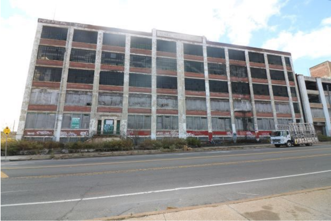
Figure 5: Plant, North (W. Allegheny Ave.) Elevation, view looking south.
