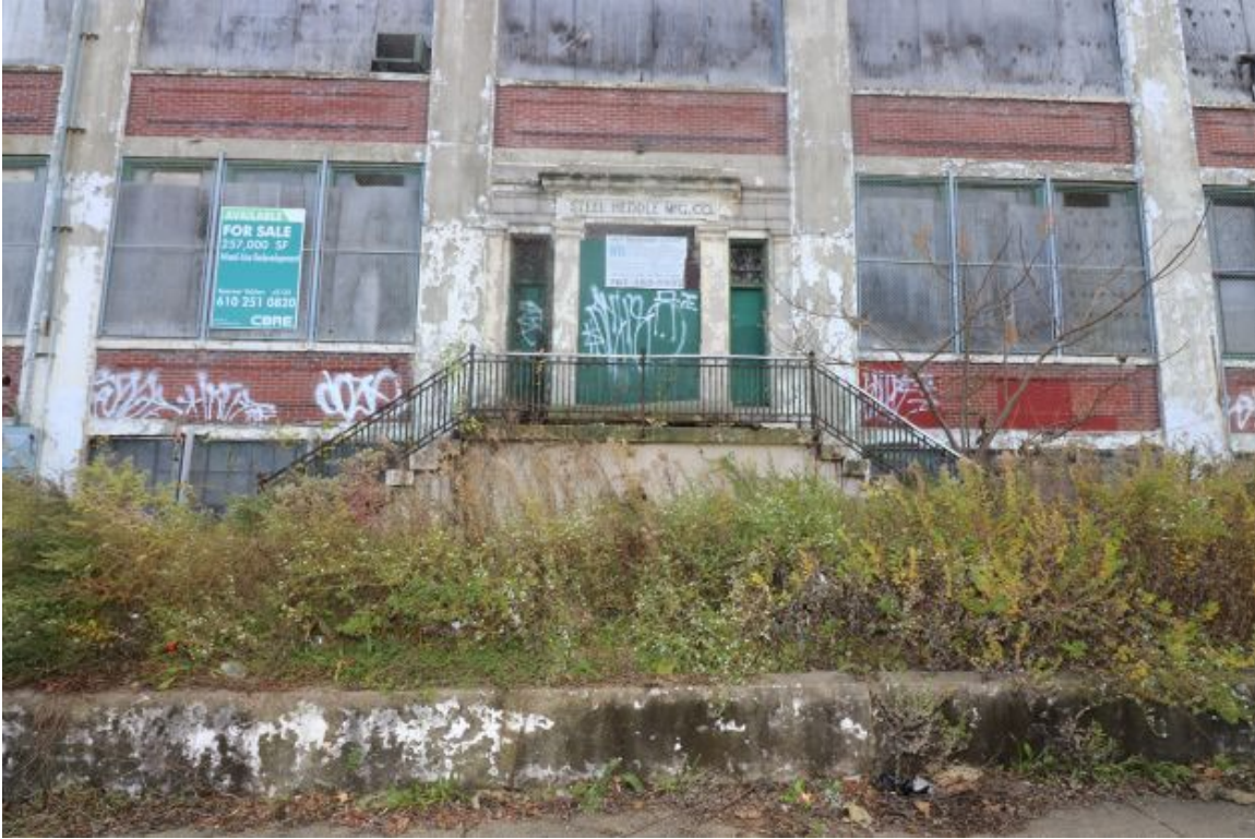
Figure 6: Plant, Primary Entrance, view looking south.
