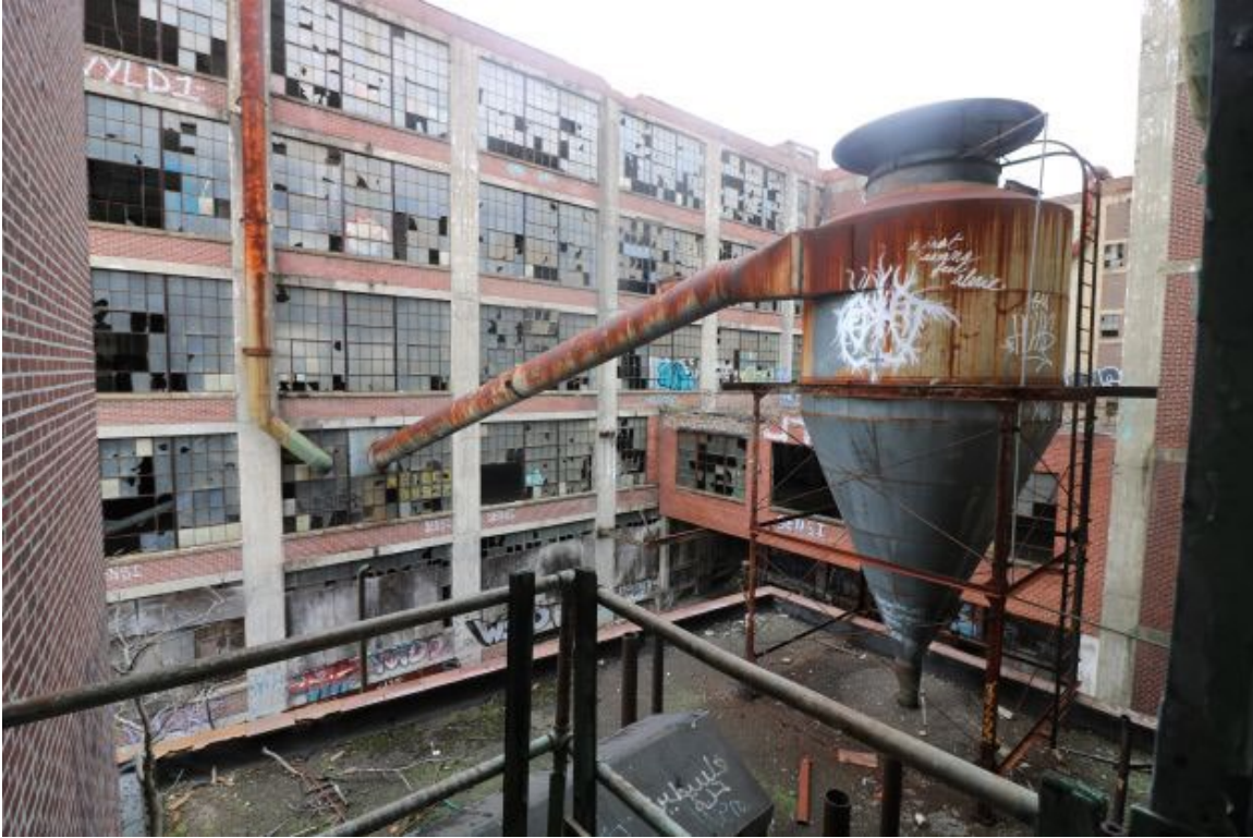
Figure 10: Plant, Courtyard, view looking northwest.
