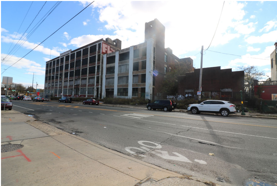
Figure 13: Chrome Plating Building, North (W. Allegheny Ave.) Elevation, view looking south.
