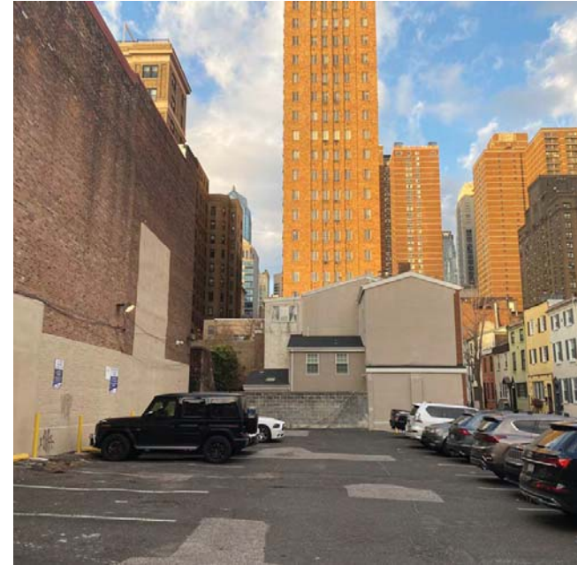
(3) VIEW OF EXISTING SITE FROM PINE ST
