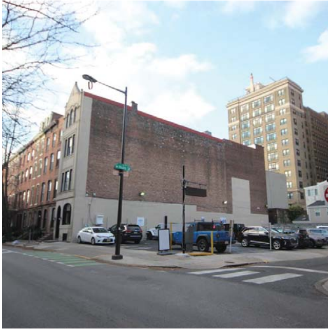
(4) CORNER VIEW FROM WEST ON PINE ST
