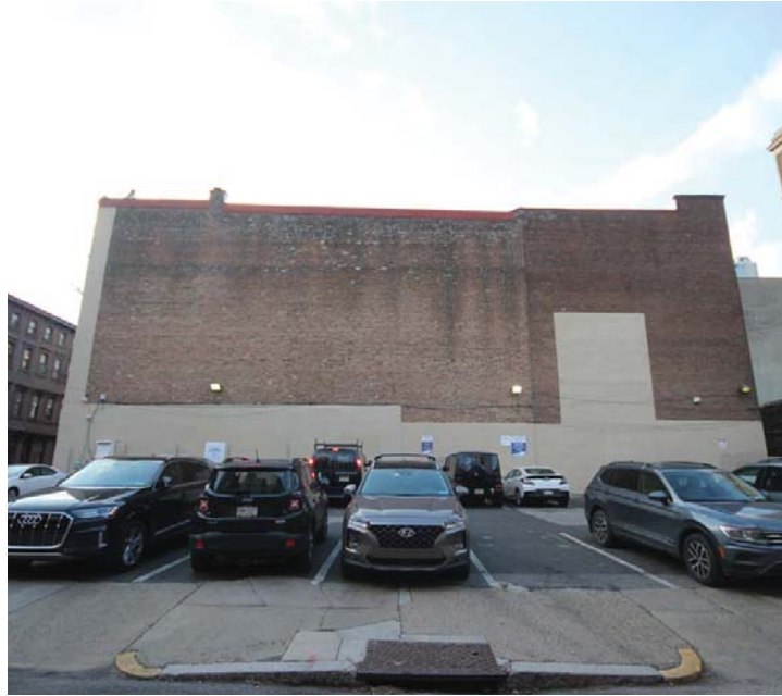
(5) VIEW WEST FROM HICKS
