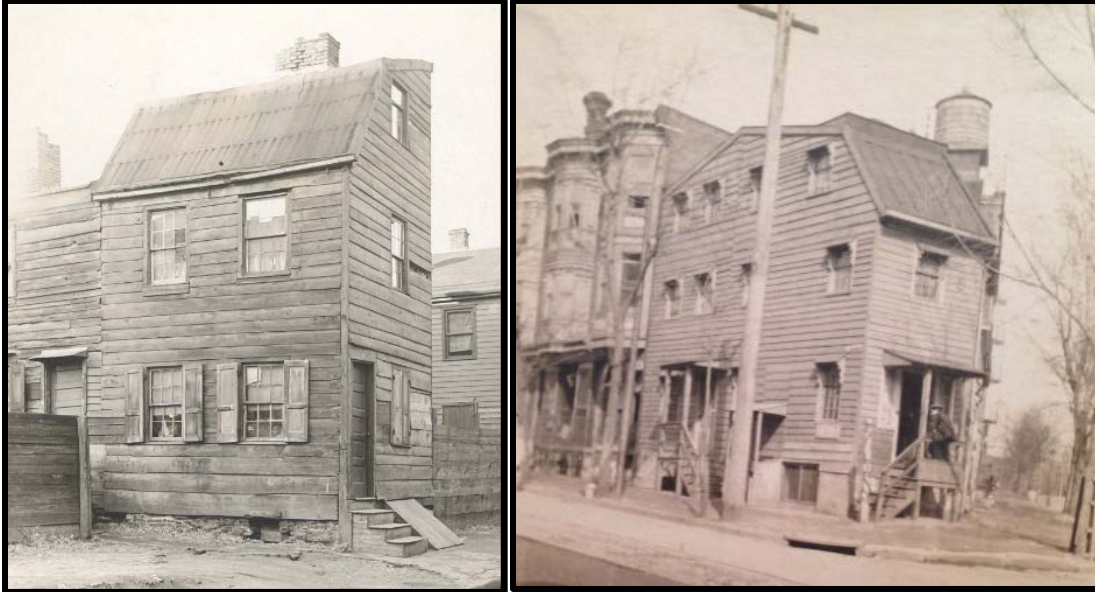
Figure 13. Left: A frame “flounder” in South Philadelphia, which, like the subject property, features a roof form defined by a broken pitch. Source: The Library Company of Philadelphia. Figure 14. Right: A wooden house with a gambrel roof at Wylie and 19 th Streets in the Francisville section of Philadelphia. Source: Perkins Collection, Historical Society of Pennsylvania.
