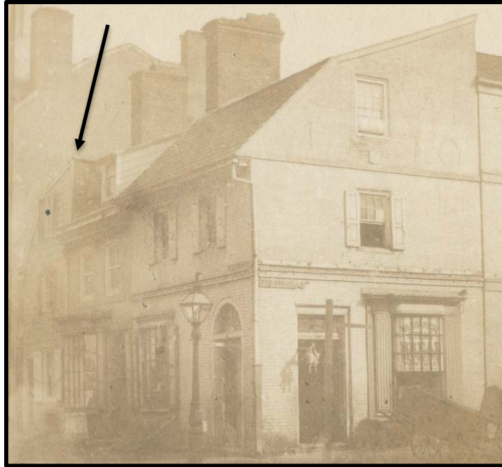
Figure 11. Still standing at the southeast corner of S. Fifth and Locust Streets, the building at the corner features a side-gabled roof in a broken pitch, gambrel form. While this brick house is similar to the subject property, its near neighbor, just two doors down (see black arrow), is perhaps identical in material composition and general appearance. Source: Library Company of Philadelphia.
