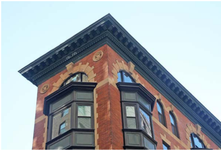
Photo 3 – Close-up detail of the cornice, windows and ornamentation at the northwest corner of the sixth and seventh floors, looking southeast from 13 th and Chestnut (Kevin McMahon, November 2021).
