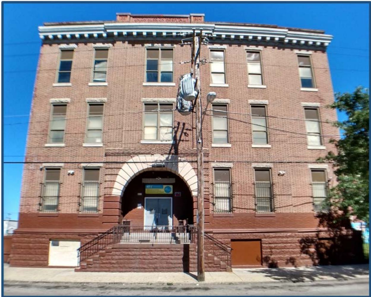
Figure 6: West façade along 4 th Street. All current photos by Steven Peitzman unless otherwise noted. The slight curvature results from the need to use a wide-angle lens. See also a Google image in the appendix.
