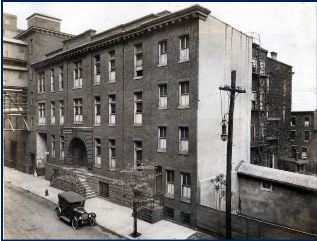
Figure 7: The nominated building from a 1919 photograph, looking north and east. The addition to the right (south) was a nurse's residence, since demolished. To the north (left) is a two-story connector that attached the hospital to a Stetson warehouse building. It was demolished in 1978.
