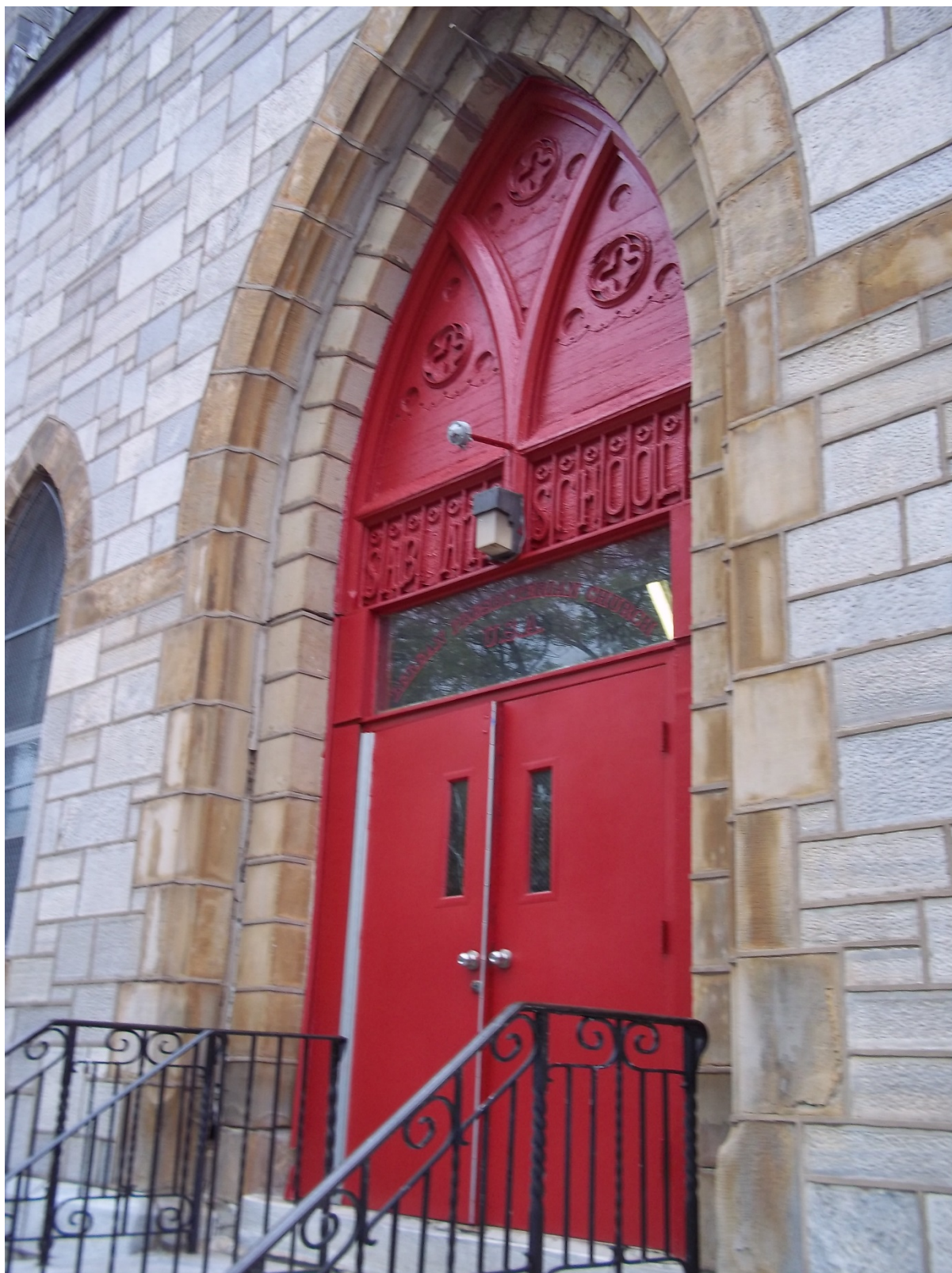
Figure 19: South side of the Sabbath School on Diamond Street. The red metal fire doors have a plate glass transom window above. The words SABBATH SCHOOL are also visible as well as three quatrefoils.
