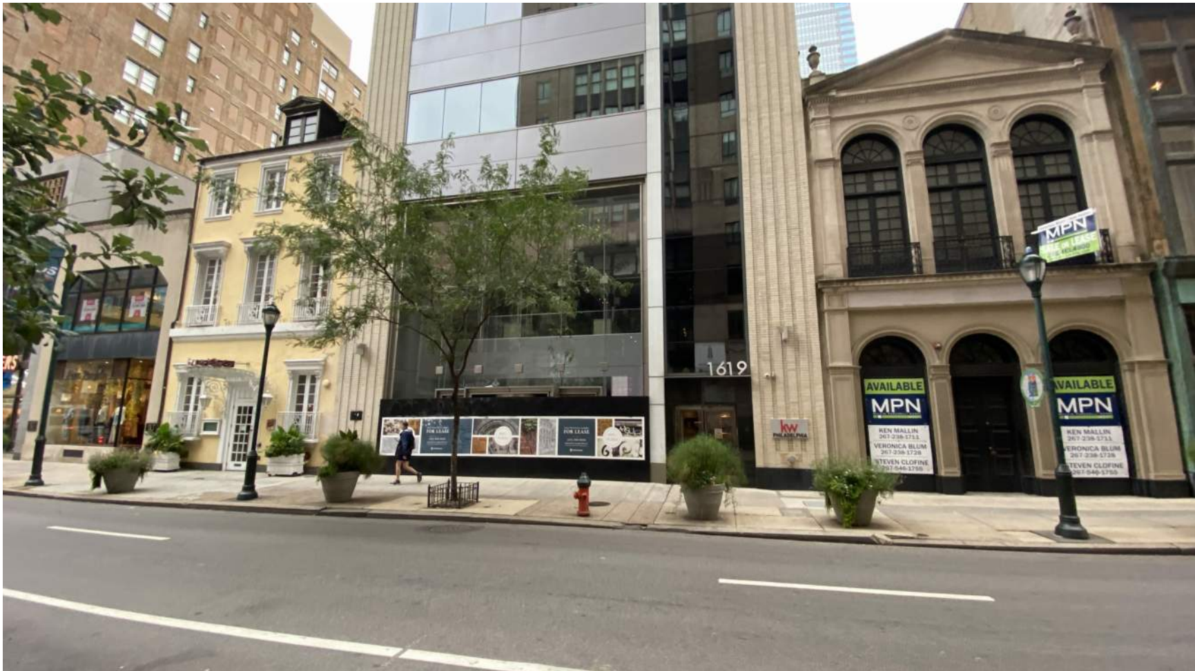
VIEW OF 1617 WALNUT ST AND BUILDINGS TO THE LEFT
