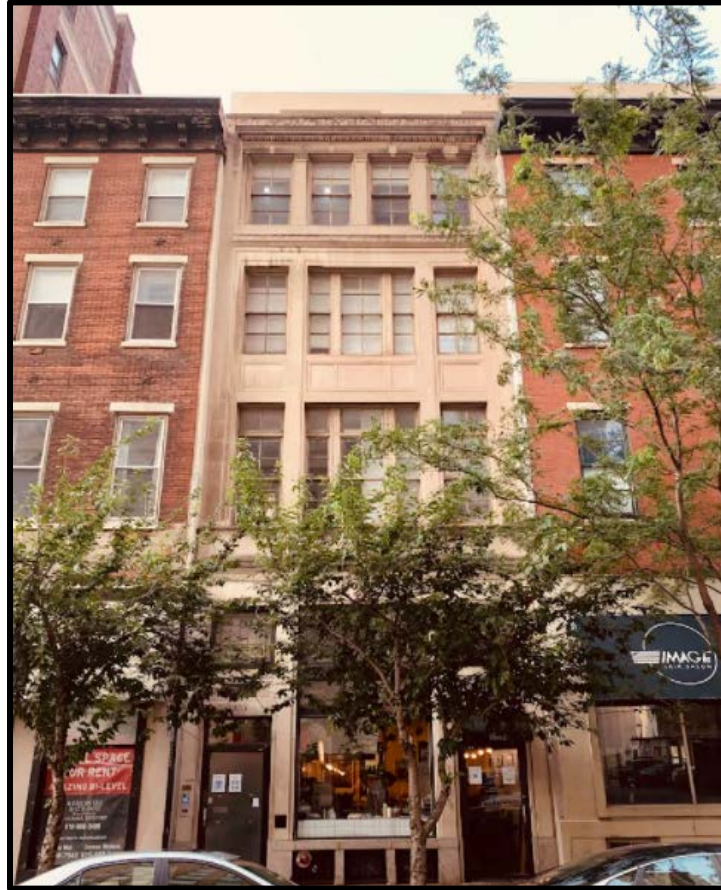
Figure 1. The primary (south) elevation. Source: Oscar Beisert, 2021.
