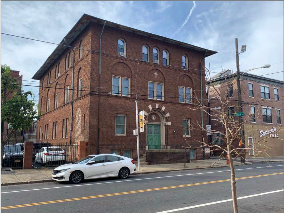
View of front (north) and east elevations.
