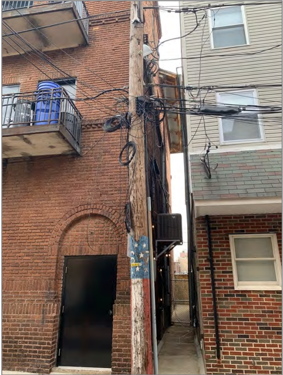
Small alleyway runs along south elevation.
