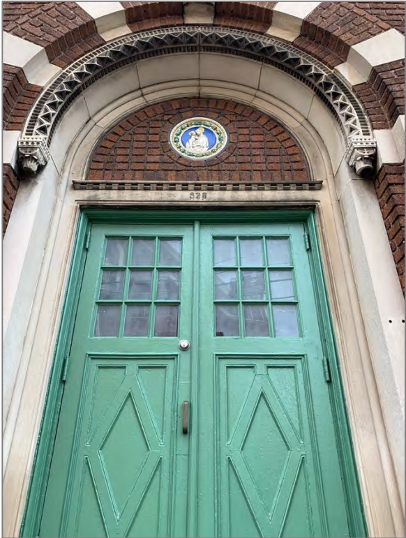
Front entryway with masonry detailing.
