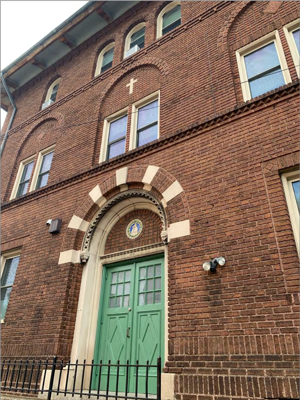
View of with main entrance and masonry details.
