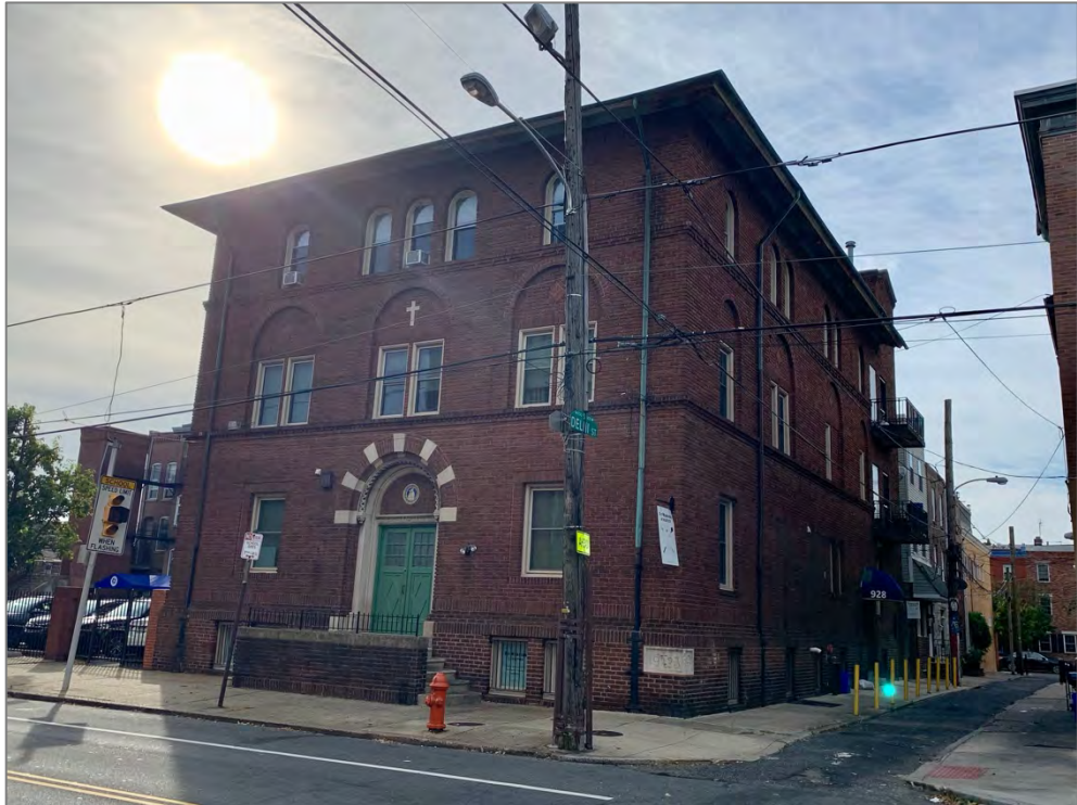
View of front (north) and west elevations. The west elevation faces S Delhi Street.
