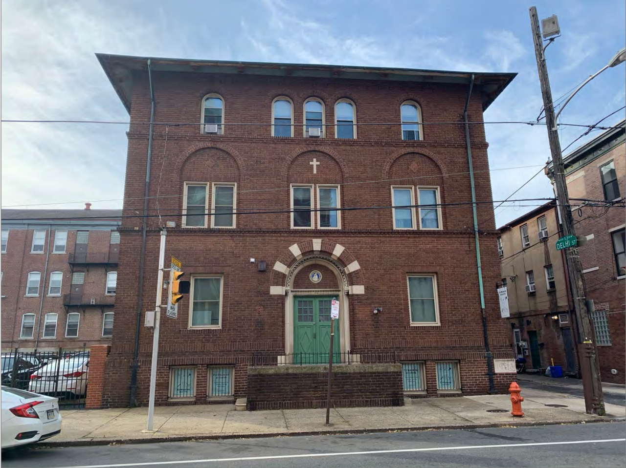
928-30 Christian Street: Front elevation along Christian Street.
