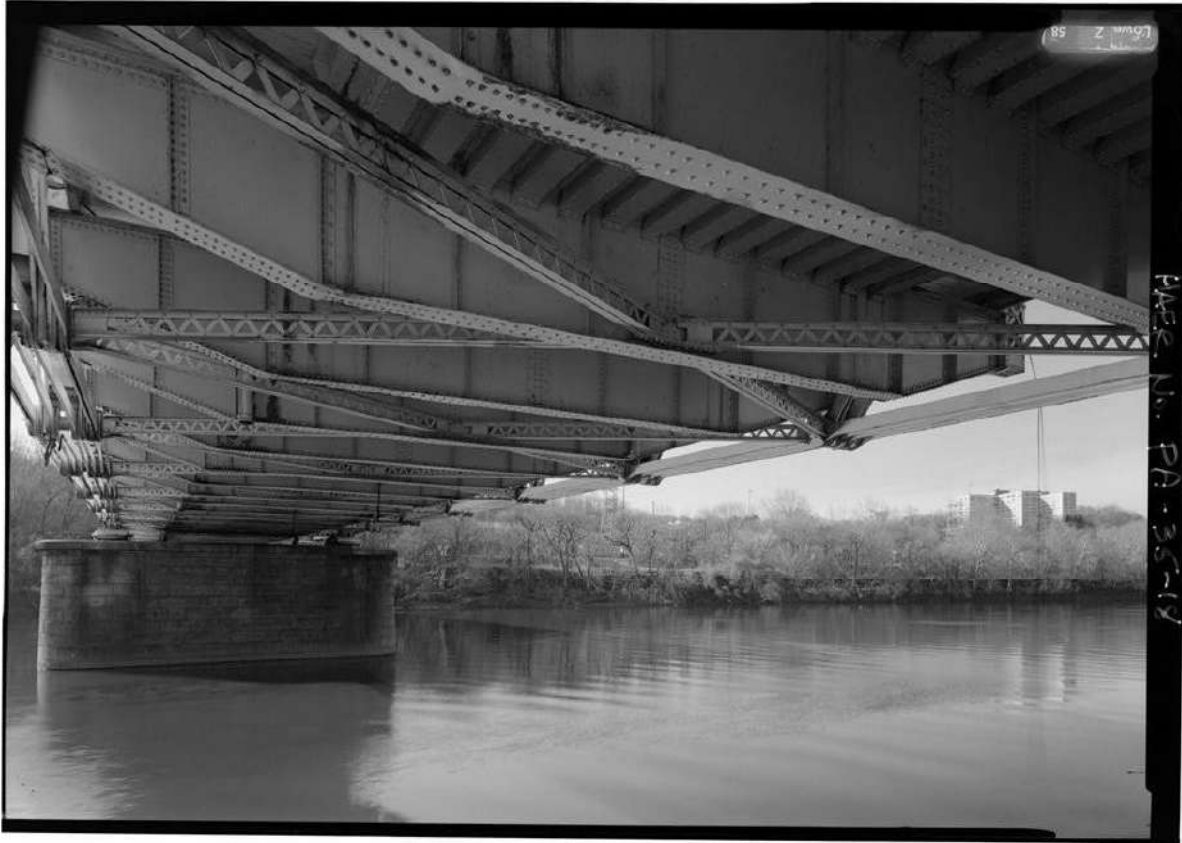
Figure 4: Image showing the tapered transverse floor beams and one of the two masonry piers which supports the bridge. Source: Falls Bridge HAER PA, 51-PHILA, 701--18.
