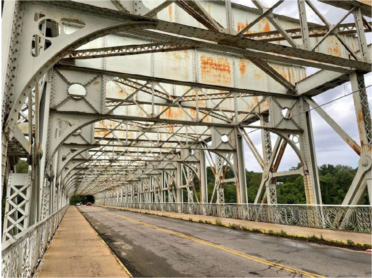
Figure 5: View from a sidewalk on the bridge which showcases the upper deck floor beams, sway bracing, and the spandrel brackets. Source: Photograph taken by Dorothy Fitzgerald, June 8, 2021.
