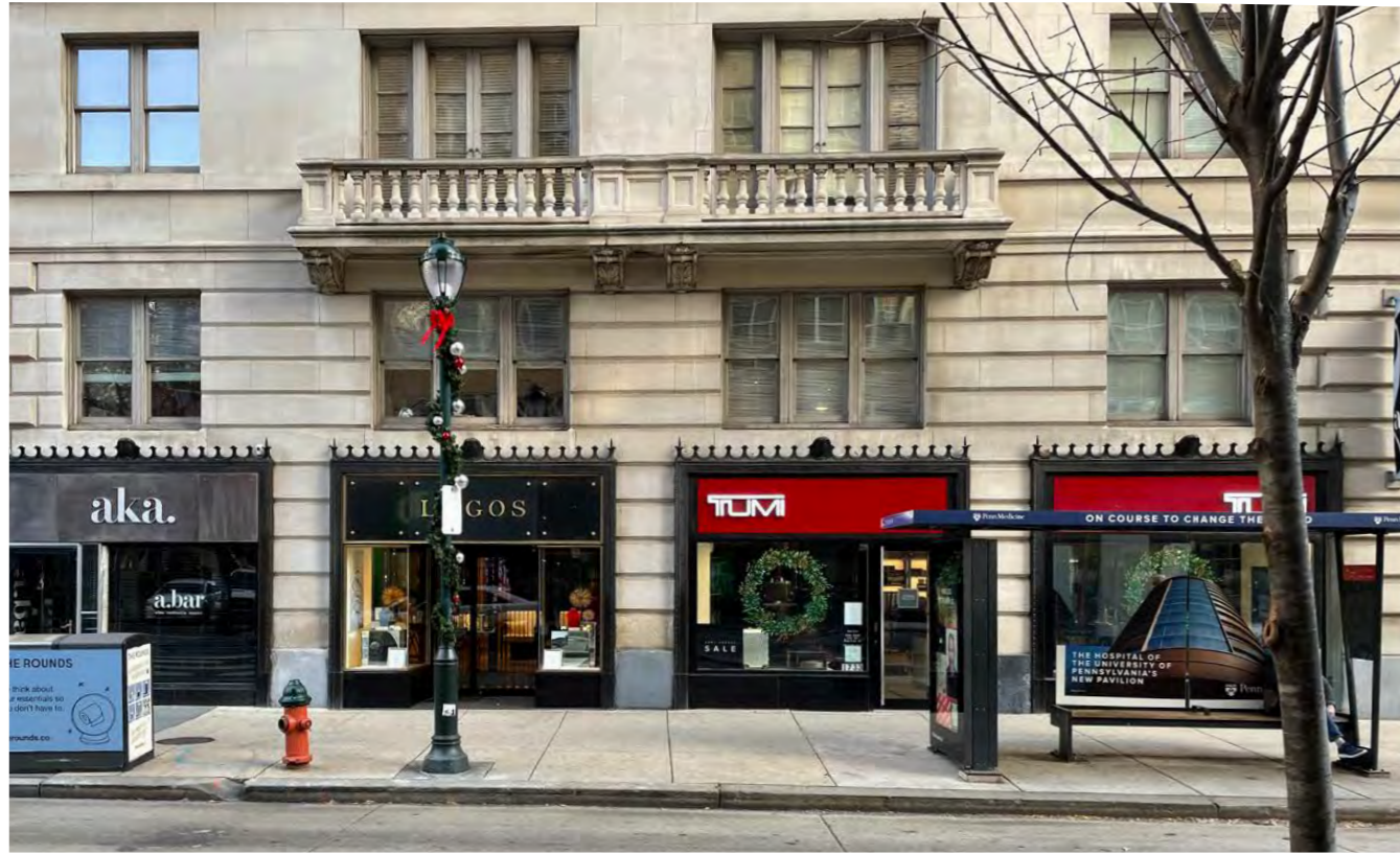
Existing: Facade to the west at the corner of 18th & Walnut Street
