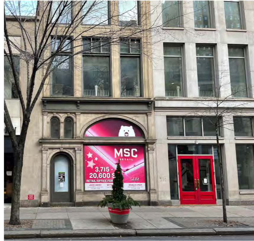
Existing: Facades to the East on Walnut Street (1715 - 1721)
