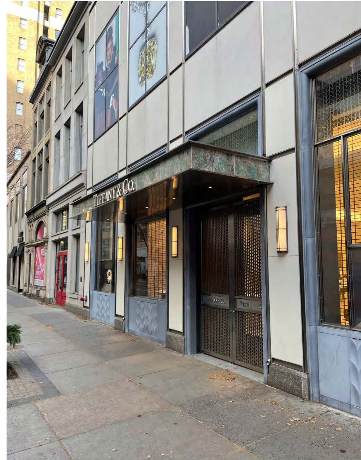
Existing: Tiffany & Co. Marquee, 1715 - 1717 Walnut Street
