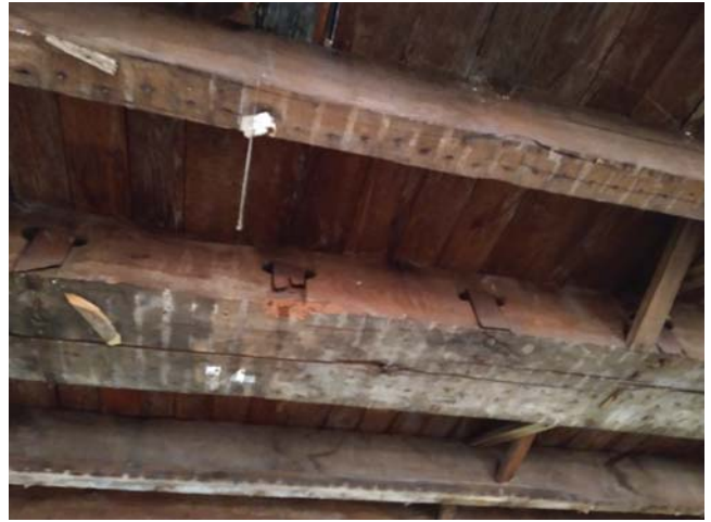
DETAIL OF SUMMER BEAM WITH TENON CUTS
