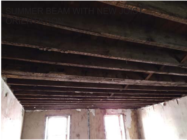
SUMMER BEAM WITH NEW JOIST ORIENTATION
