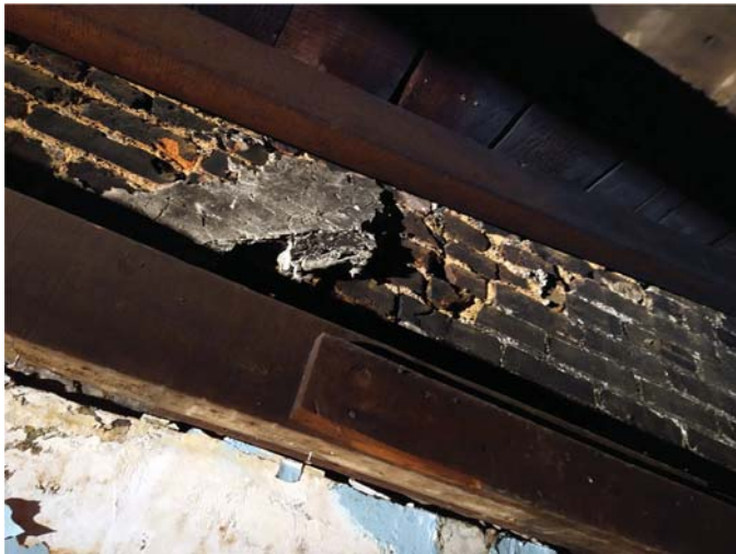
EVIDENCE OF GARRET ROOF AT 312
