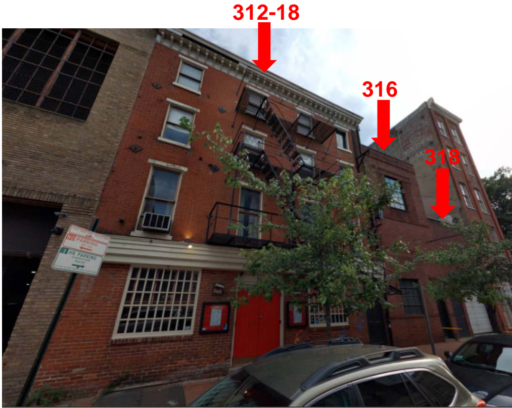
Figure 2: 312-14, 316, and 318 Race Street, 2019. Source: Cyclomedia.
