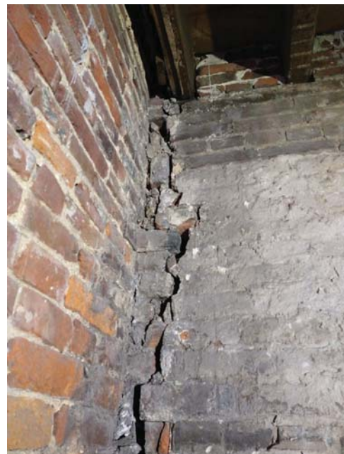
DETAIL OF COLD CONNECTION
