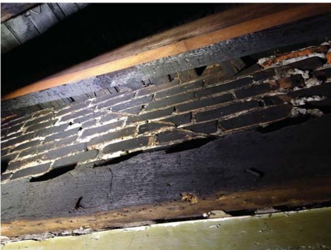
EVIDENCE OF GARRET ROOF AT 314
