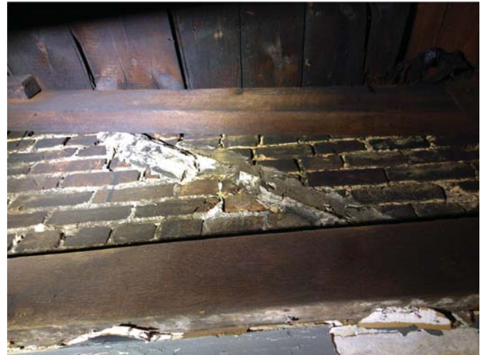
EVIDENCE OF GARRET ROOF AT 312
