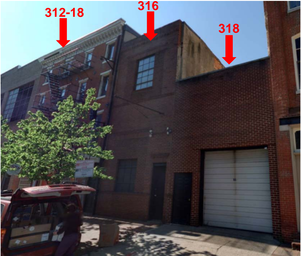
Figure 3: 312-14, 316, and 318 Race Street, 2019. Source: Cyclomedia.
