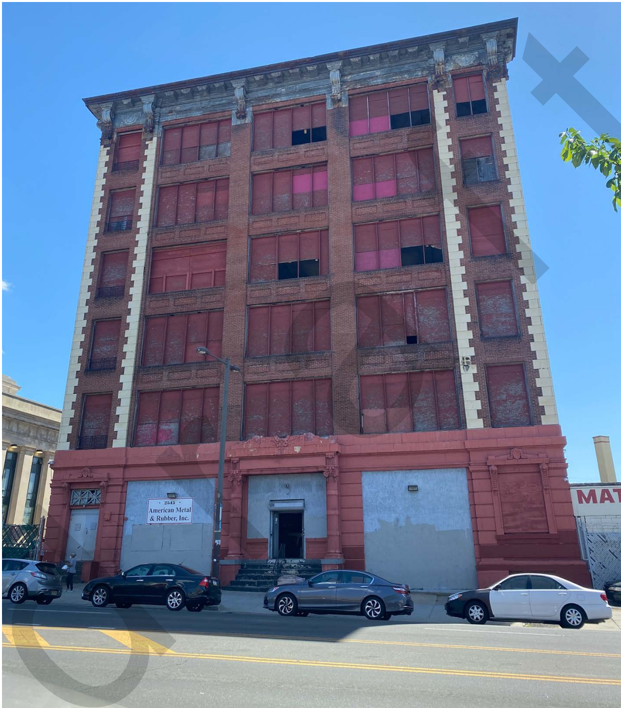
Photograph 1 – West elevation, view east
