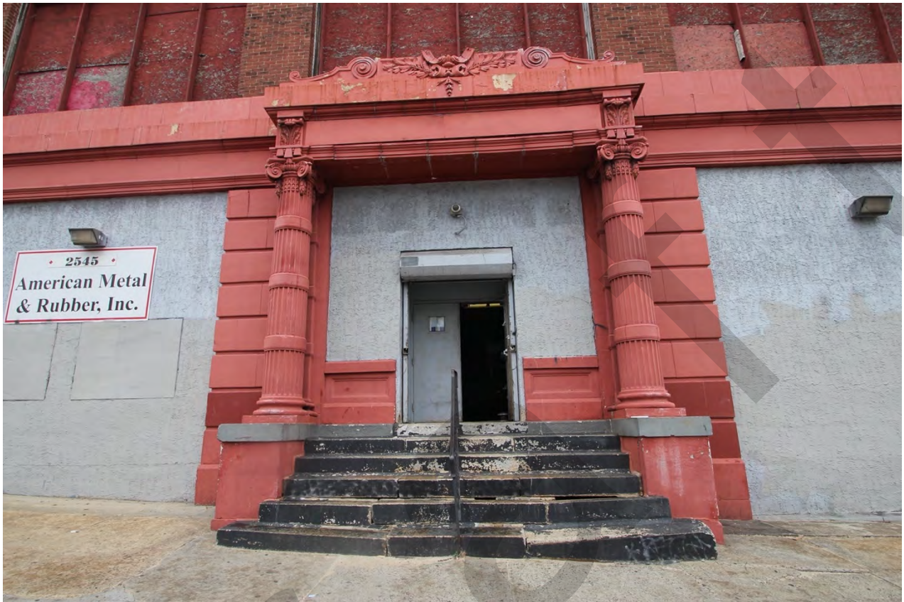
Photograph 3 – West elevation, Entrance detail, view east. Note the terra cotta detailing by the Conkling Armstrong Terra Cotta Company.
