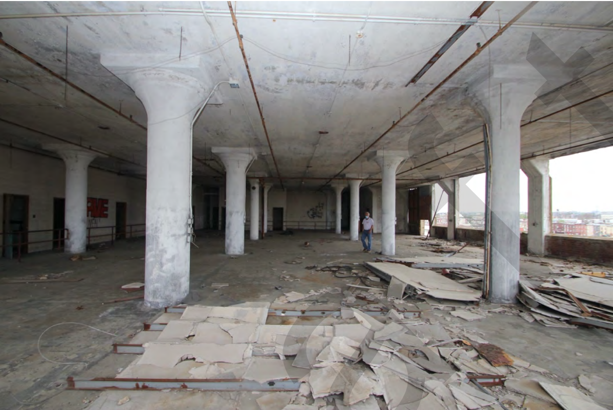
Photograph 20 – 5th floor, view east
