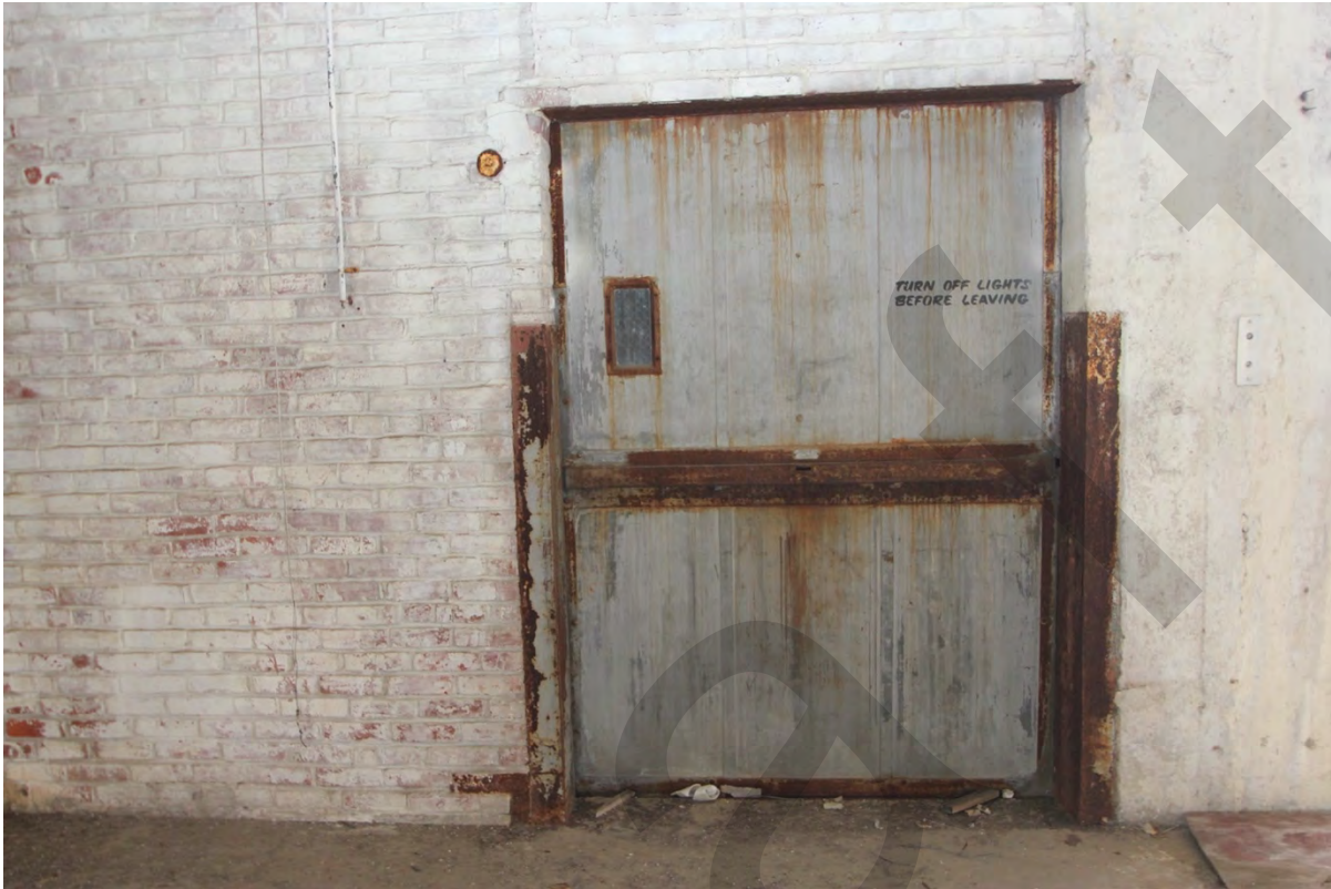
Photograph 18 – 4th floor, Elevator, view north
