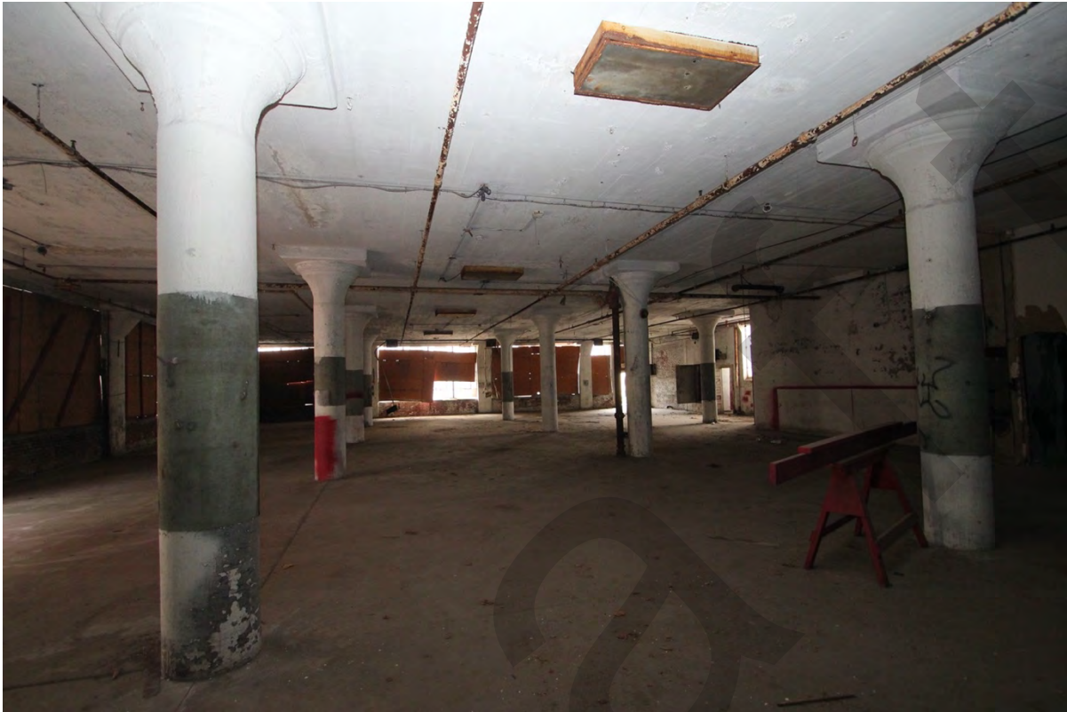
Photograph 11 – 2nd floor, view west
