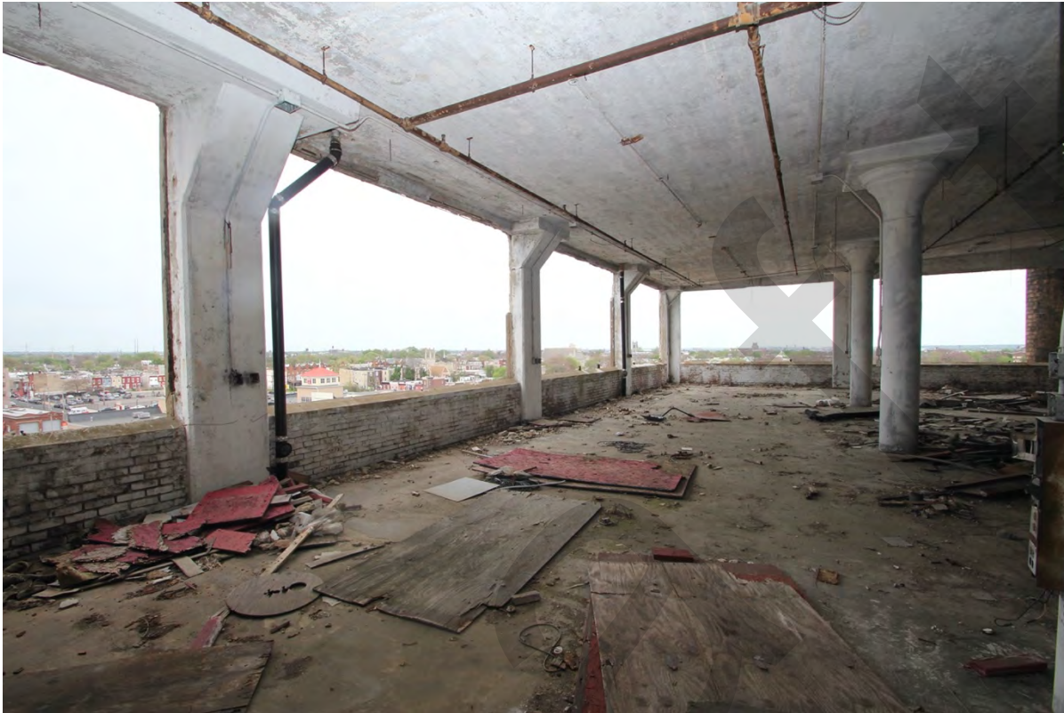
Photograph 24 – 6th floor, view east
