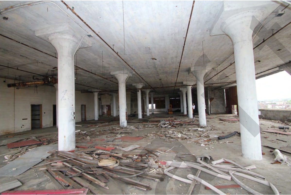
Photograph 22 – 6th floor, view east
