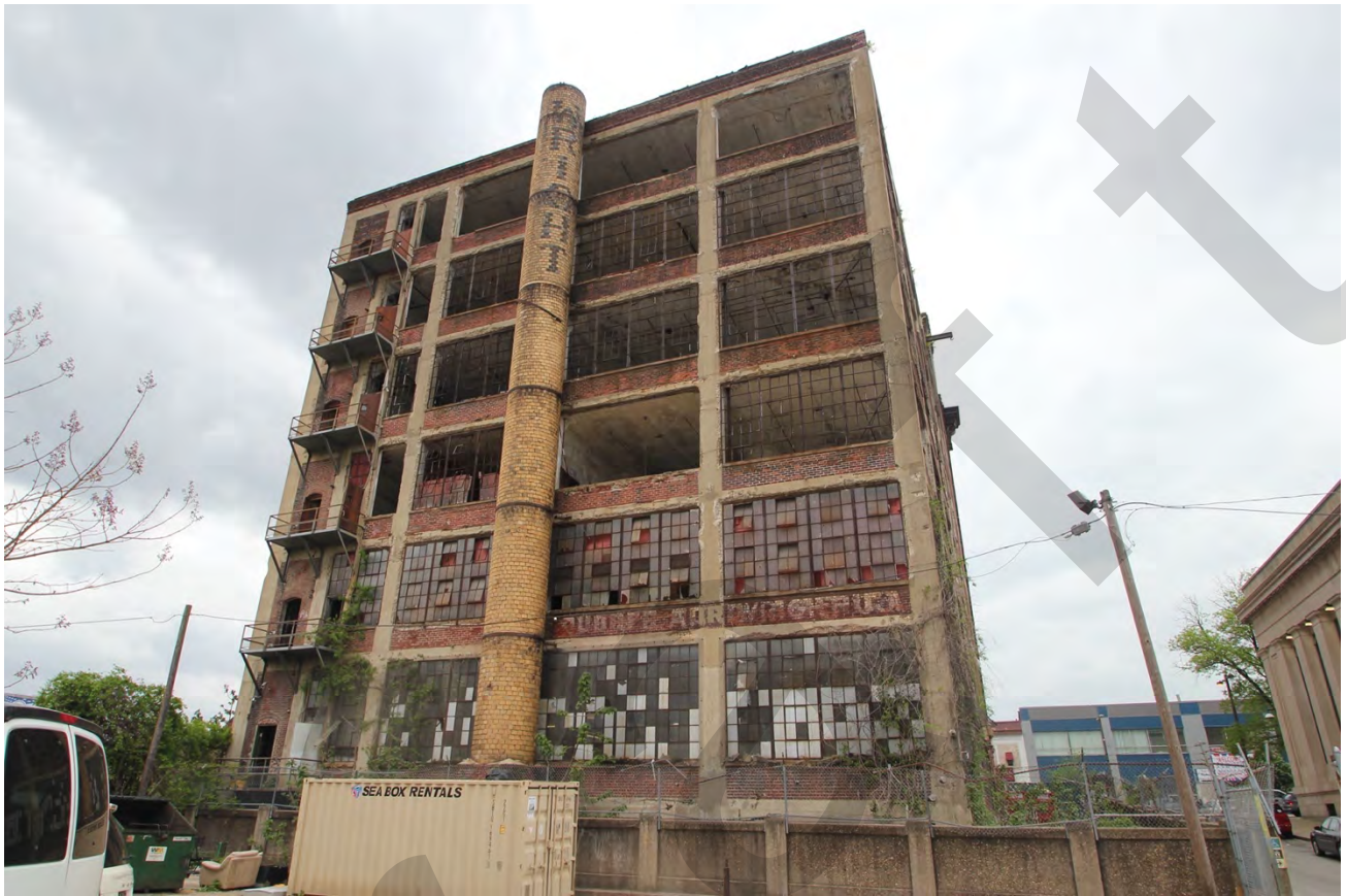
Photograph 6 – East elevation, view southwest
