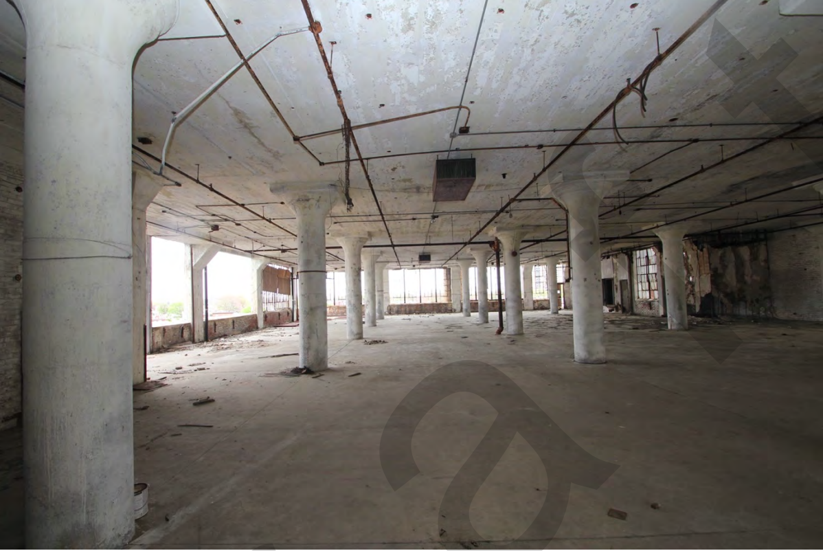
Photograph 14 – 3rd floor, view east
