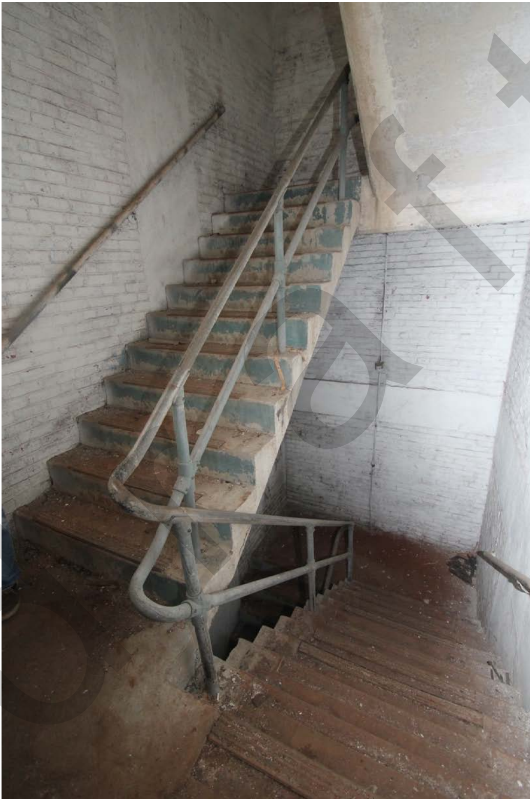
Photograph 13 – 2nd floor, Stairway, view west
