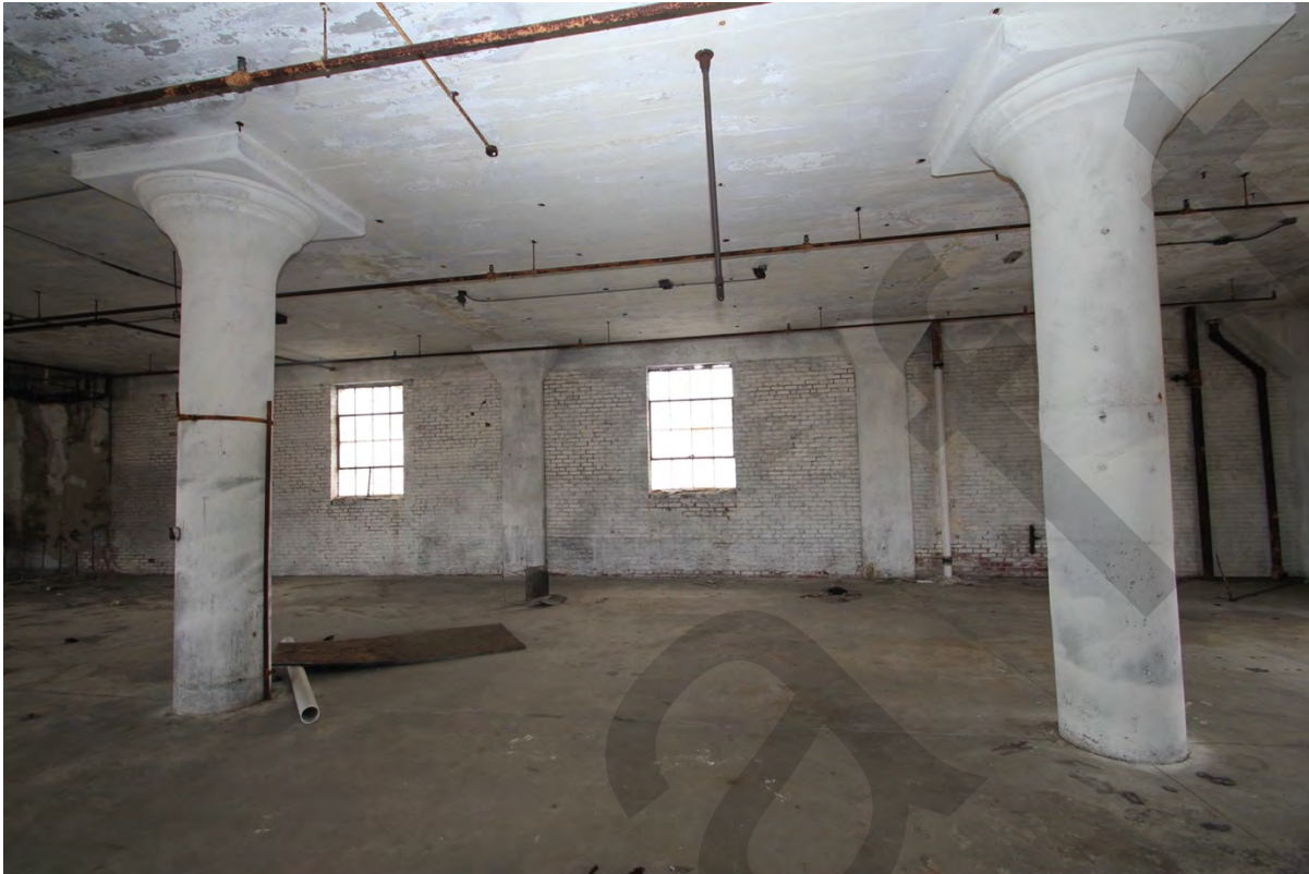
Photograph 17 – 4th floor, view south
