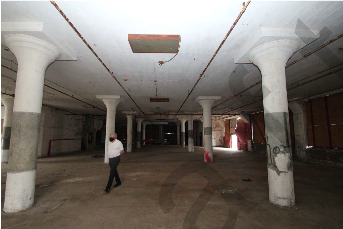
Photograph 12 – 2nd floor, view east
