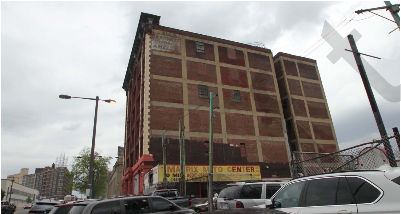
Photograph 5 – West and south elevations, view northeast
