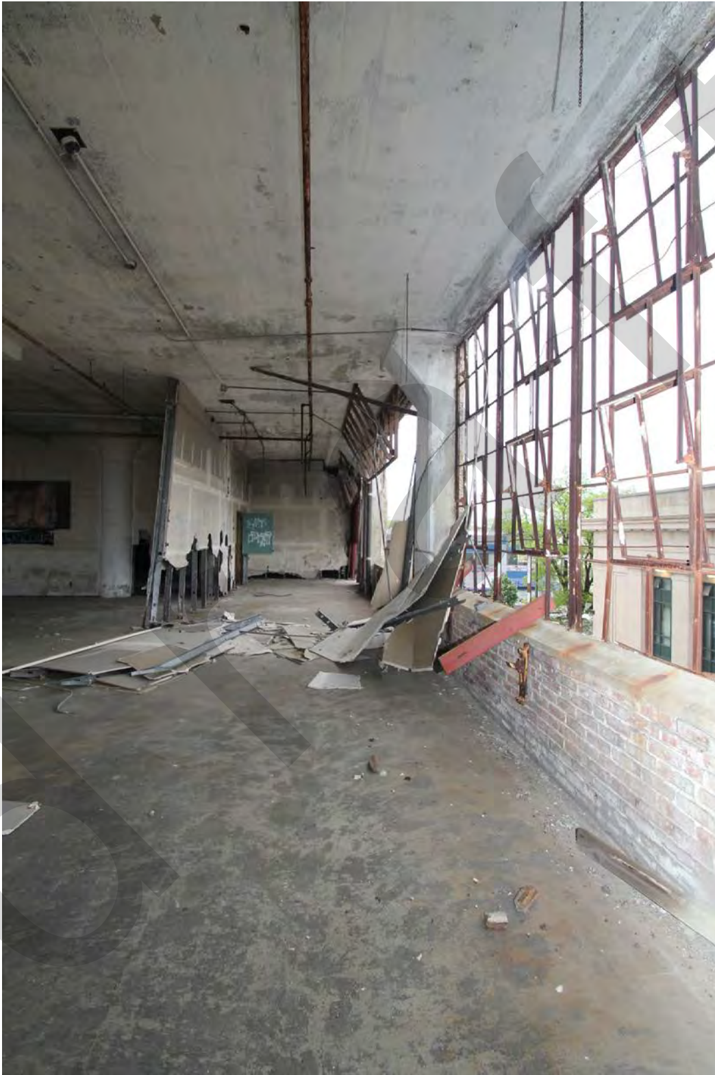
Photograph 16 – 3rd floor, view west
