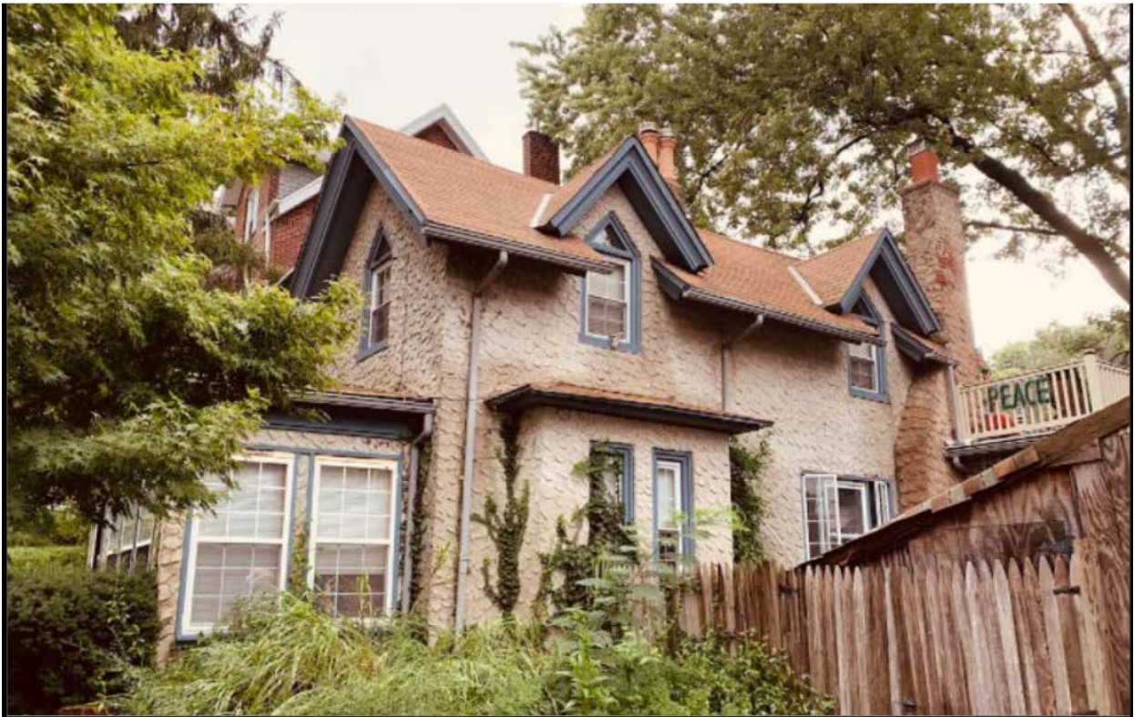
Figure 5: Northwest and southwest elevations; photo from nomination, 2021. Source: Historical Commission files.
