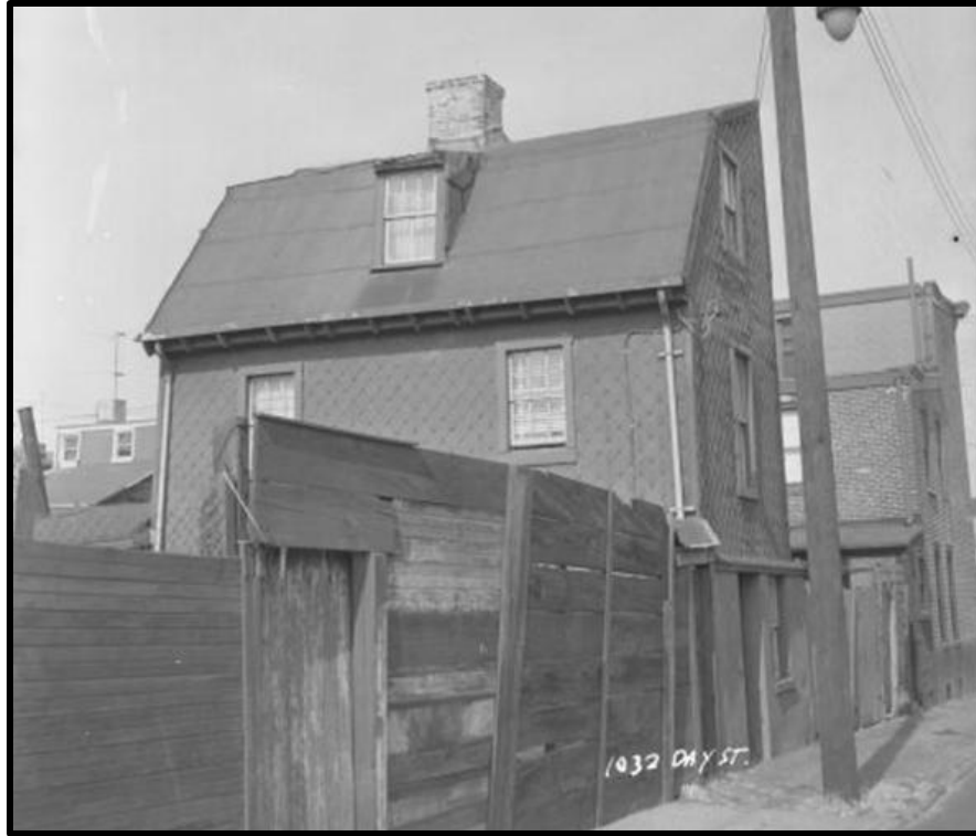
Figure 1 (repeated). The side (east) and primary (north) elevations of the subject property in 1958. Source: Phillyhistory.org.
