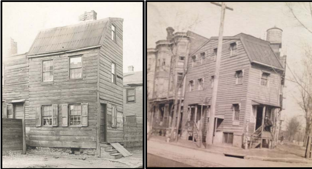
Figure 13. Left: A frame “flounder” in South Philadelphia, which, like the subject property, features a roof form defined by a broken pitch. Source: The Library Company of Philadelphia. Figure 14. Right: A wooden house with a gambrel roof at Wylie and 19 th Streets in the Francisville section of Philadelphia. Source: Perkins Collection, Historical Society of Pennsylvania.
