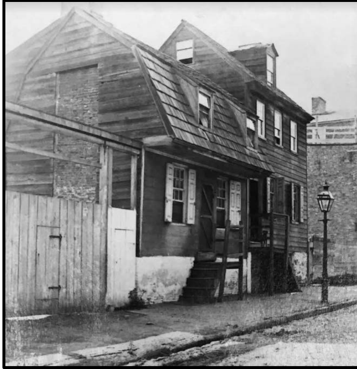
Figure 24. Frame dwellings on Warren Street in Fishtown, ca.1880-90, including the early one-and-one-half-story wooden house on left with its fully articulated side-gable, gambrel roof and shed dormer. Source: Castner Scrapbook on Old Houses, Free Library of Philadelphia. Note that the house on right is similar in form and scale to the subject property.
