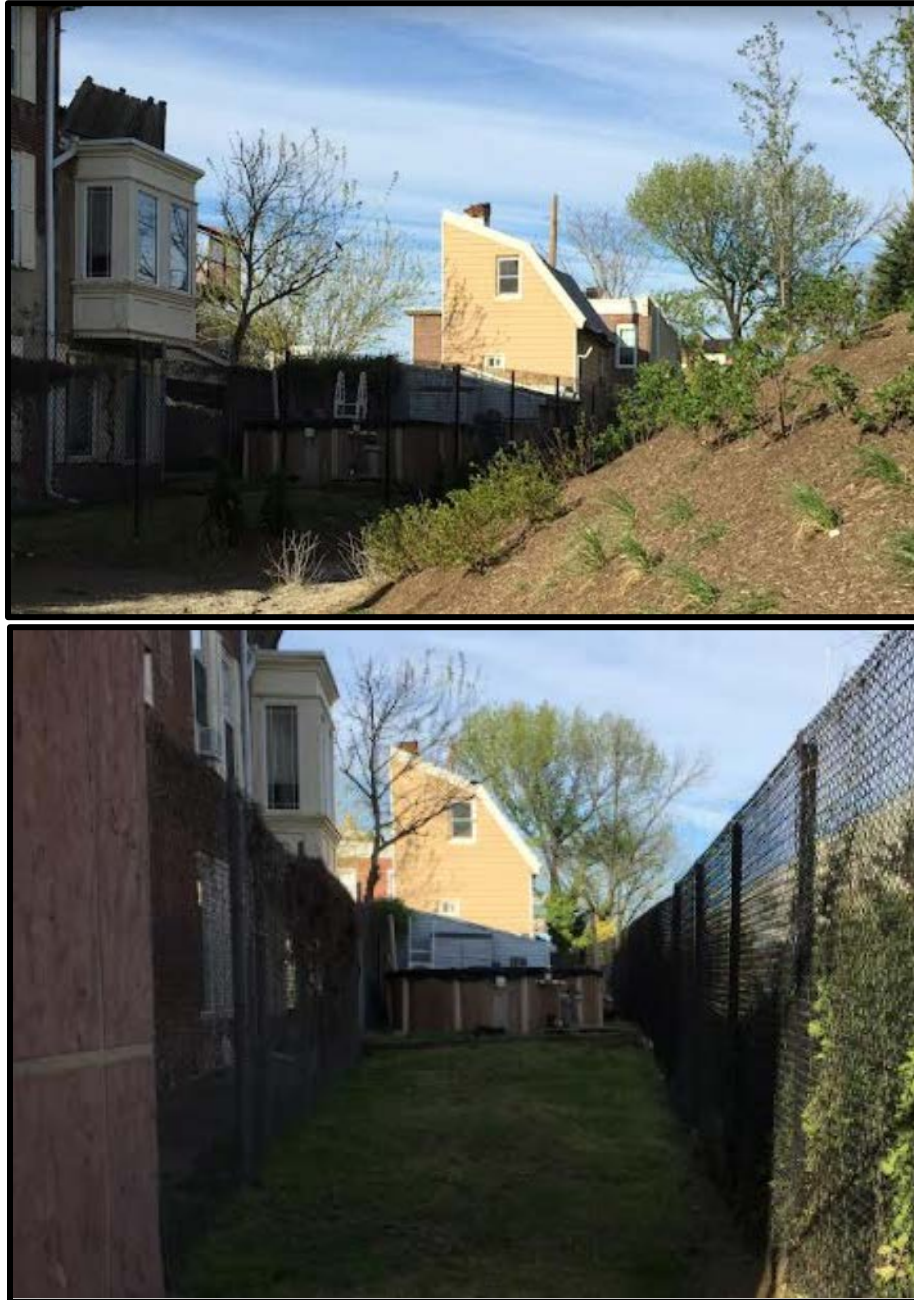
Figure 8. Top: Looking northwest at the side (east) and rear (south) elevations of the subject building. Source: Oscar Beisert, 2020. Figure 9. Bottom: Looking north at the rear (south) elevation of the subject building. Source: Oscar Beisert, 2020.
