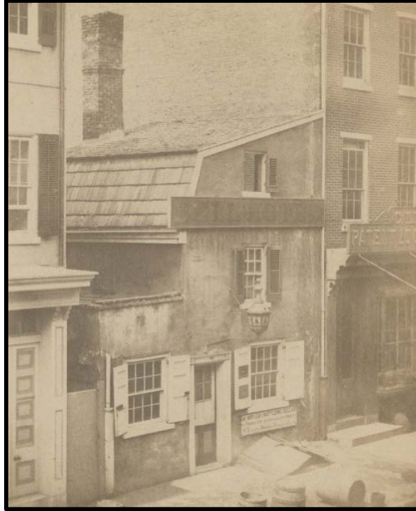
Figure 10. The Bell Tavern was a "flounder," like the subject building, that once stood on the west side of Eighth Street north of Sansom. This "half-house" and its gambrel roof was demolished in 1858. This photograph was taken by Richards in 1857. Source: The Library Company of Philadelphia.
