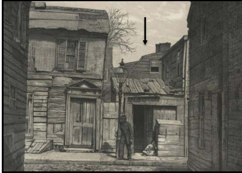
Figure 19. Seen between like wooden houses, the Georgian doorway in the lithograph is what remains of this like-style dwelling. In the background on right is a wooden house with a gambrel roof. This is on a whole a court of wooden houses depicted in The little homeless one or “no one to kiss me good night.” Lithograph by P.S. Duval, Philadelphia, 1867. Courtesy the Library Company of Philadelphia.
