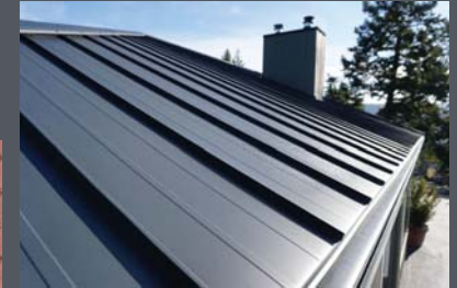
11" Standing Metal Seam Roof Dark Taupe or Grey to match wood exterior
