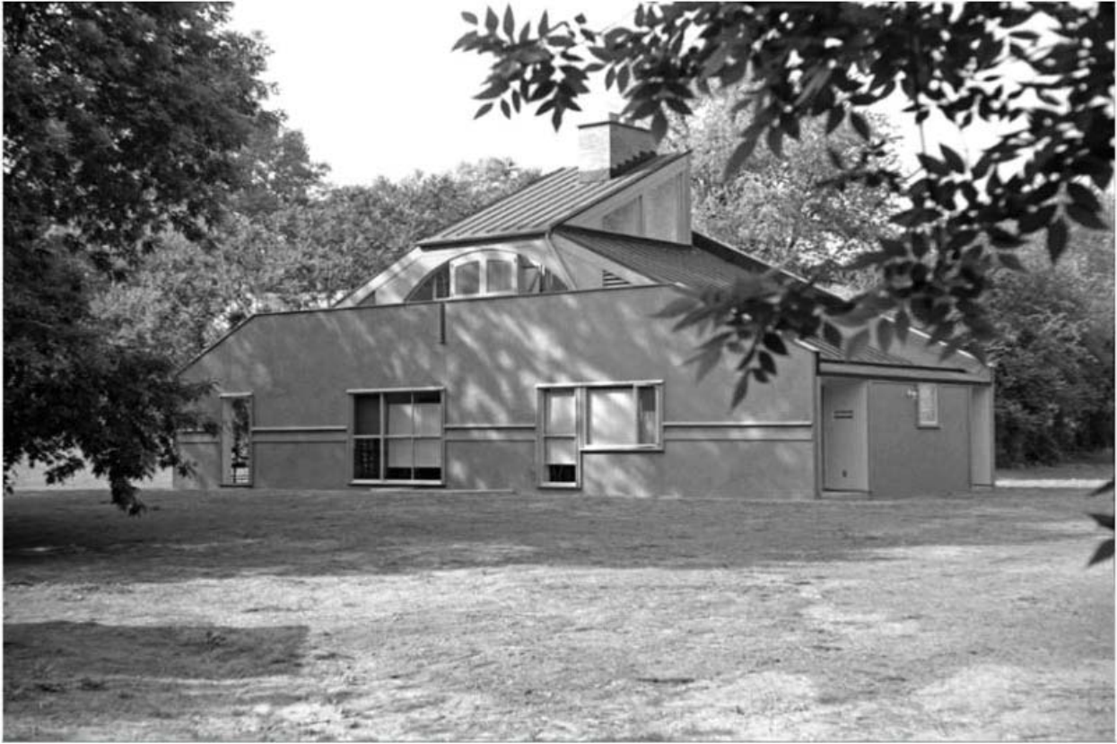
Figure 6: Historic photo of the rear elevation, undated. Source: Historical Commission files.
