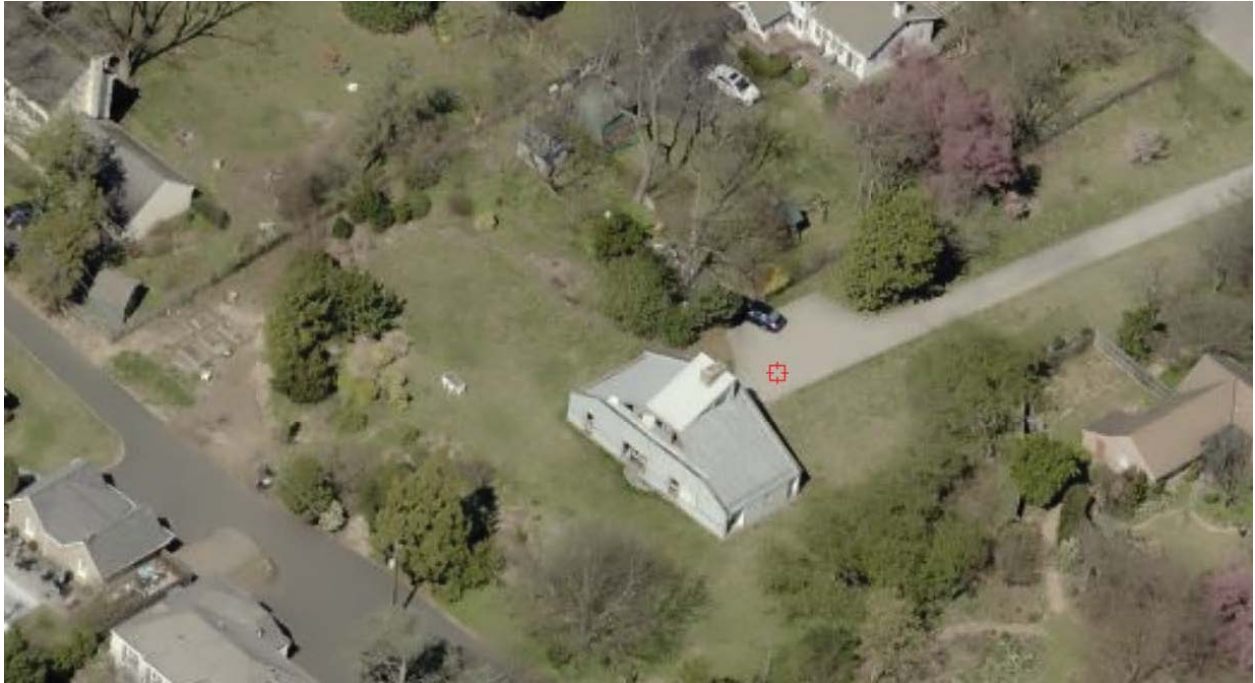
Figure 4: Rear of 8330 Millman Street, 2020. Source: Pictometry.
