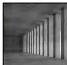
⑤ CONCRETE COLUMNS
