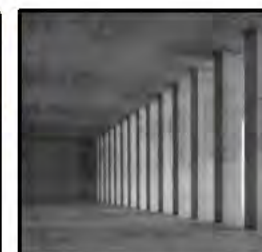
⑭ CONCRETE COLUMNS
