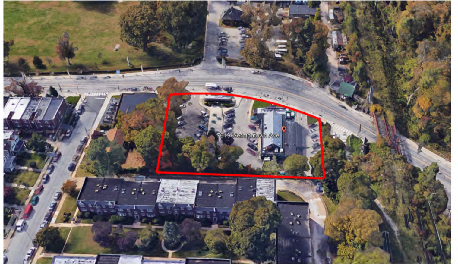
EXISTING AERIAL 2 - SOUTH
