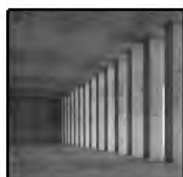
⑤ CONCRETE COLUMNS
