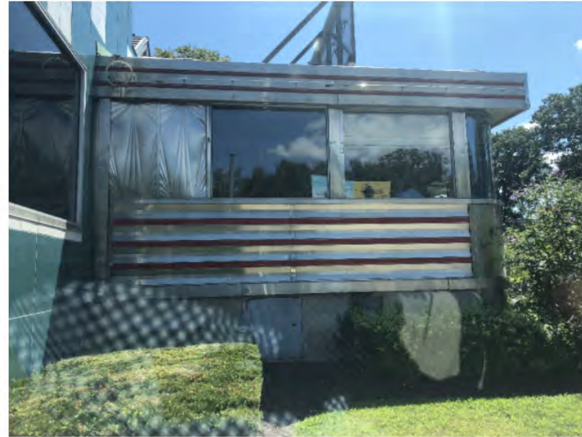
SITE PHOTO 3: LOOKING AT WEST SIDE OF EXISTING BUILDING
