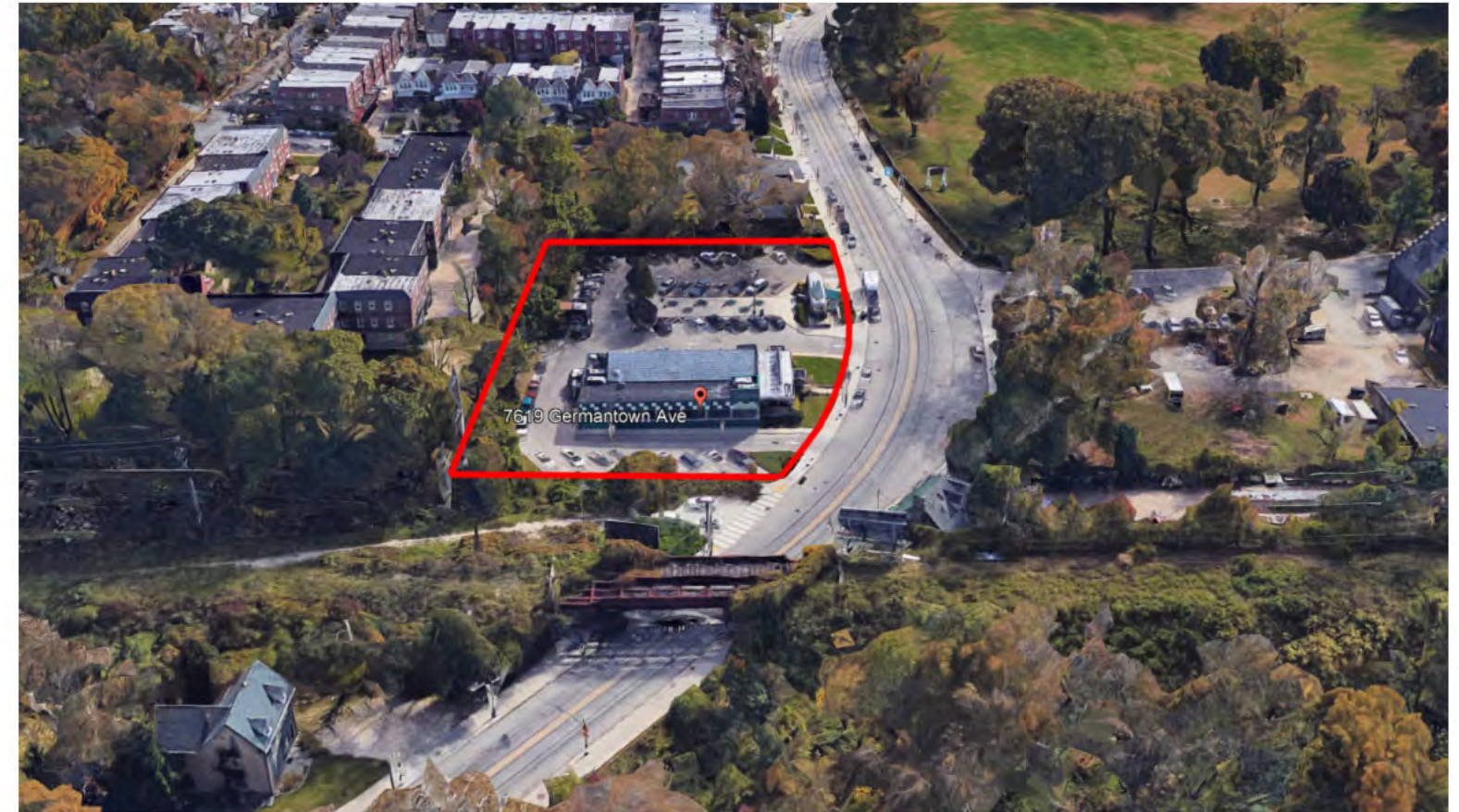
EXISTING AERIAL 4 - EAST
