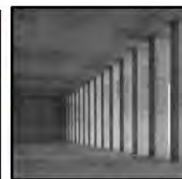
⑤ CONCRETE COLUMNS
