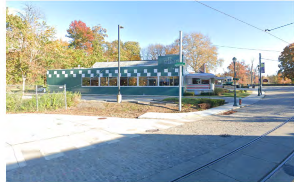
SITE PHOTO 5: LOOKING SOUTH - EAST AT EXISTING BUILDING
