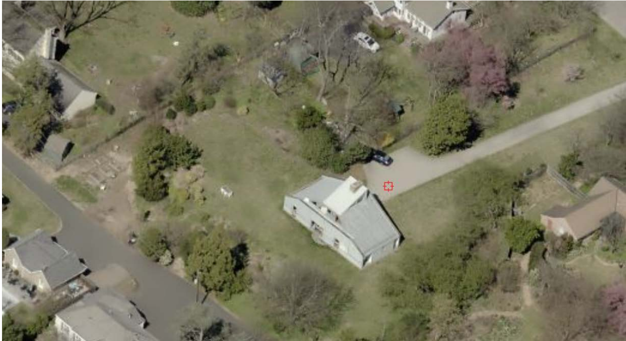
Figure 4: Rear of 8330 Millman Street, 2020. Source: Pictometry.
