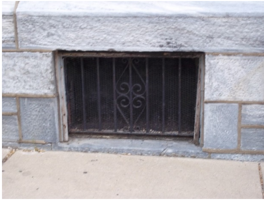
Figure 17: South side of the Sabbath School on Diamond Street. Three basement windows are covered with black metal grates which have a curlicue design. A fourth window has been filled with glass block. Images are shown on the facade from west to east: window one (top left), window two (top right) and window three (bottom left), and window four (bottom right).
