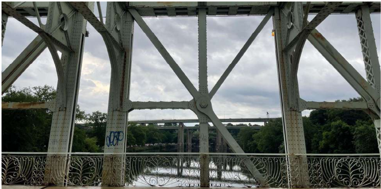
Figure 8: Truss design with auxiliary sub-struts. Source: Photograph by Dorothy Fitzgerald, June 8, 2021.
