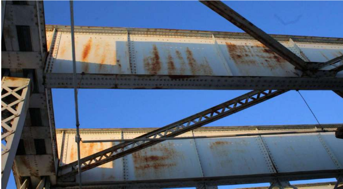
Figure 12: The floor beams for the upper deck, extending over three feet above the upper chord, seen on the left side of the image. Source: Photograph by Taryn Williams, November 14, 2020.
