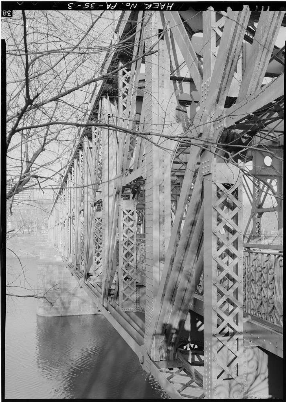
Image 11: "Truss Detail." Source: Falls Bridge HAER PA, 51-PHILA, 701--3, Prints and Photographs Division, Library of Congress.
