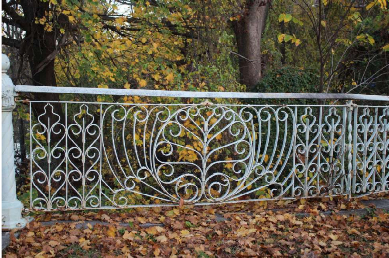
Figure 7: Wrought-iron railing and cast-iron terminal posts which are featured on both approaches to the bridge. The “tree of life” design under the railing is repeated throughout the length of the bridge. Source: Photograph by Taryn Williams, November 14, 2020.
