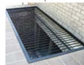
IRON GRATE LIGHT WELL COVER - PAINT BLACK SET ON 6" H CONCRETE CURB
