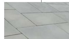
THERMAL FINISH BLUESTONE (NOMINAL 24 x 36) FOR PORCH AND RAMP
