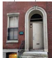
DEMO EXISTING DOOR, FAN LIGHT, AND WOOD WALL INFILL DEMO LATE 19TH CENTURY 4 OVER 4 SASH ON GROUND FLOOR
