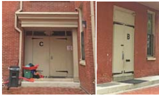
EXISTING DOORS/STRAP HINGES TO BE PRESERVED
