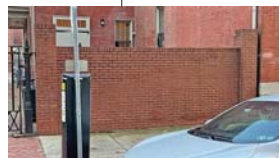
DEMO EXISTING 20TH CENTURY BRICK WALL
