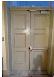
RESTORED DOORS PINNED BACK ON EXISTING STRAP HINGES AS DECORATIVE ELEMENT
