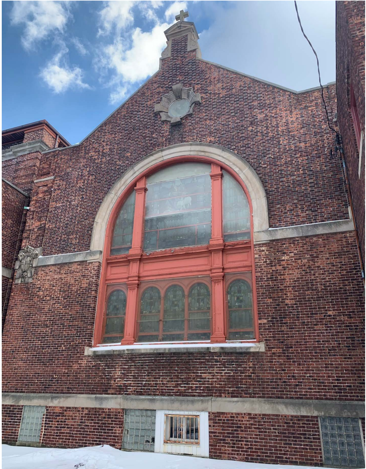
Figure 4. One of two dominant stained glass windows, this one along the Kimball Street side elevation, showing the stained glass protected behind plexiglass. February 2021.
