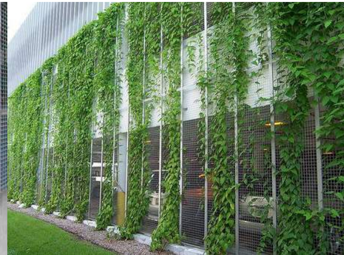
GARAGE LEVEL GRATE WITH GREENERY
