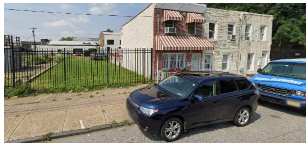
(G) 2204-2208 EAST CLEARFIELD STREET
