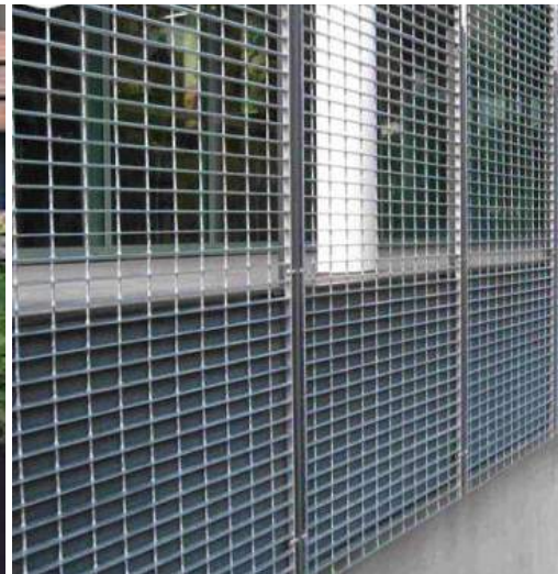
GARAGE LEVEL GRATE
