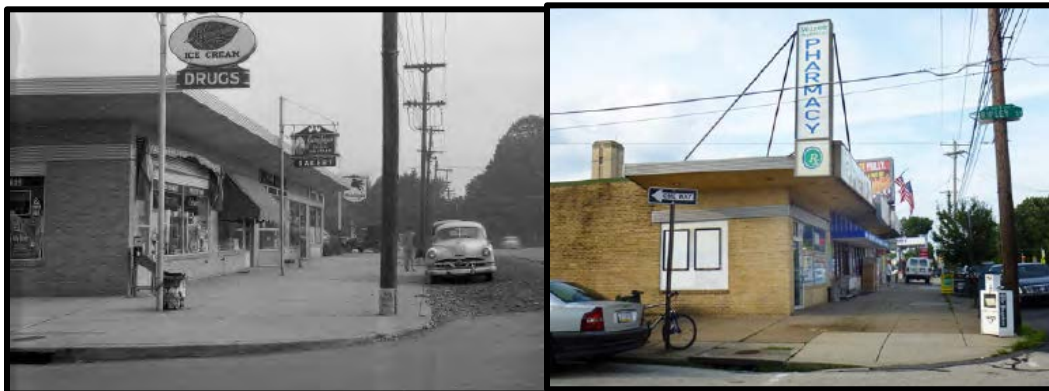
A Drug Store or Pharmacy at Verree Road and Ripley Street has maintained much of its original character. Figure 22. Left: Verree Road and Ripley Street in 1956. Figure 23. Right: Verree Road and Ripley Street in 2013. Source: Mid-Century Modern Commercial Corridors, Central Northeast District . Philadelphia City Planning Commission, 2014. http://chconservancy.org/wp-content/uploads/2017/12/MidCentury-Modern-Commercial-Corridors-CNE.pdf . Accessed 29 July 2019.
