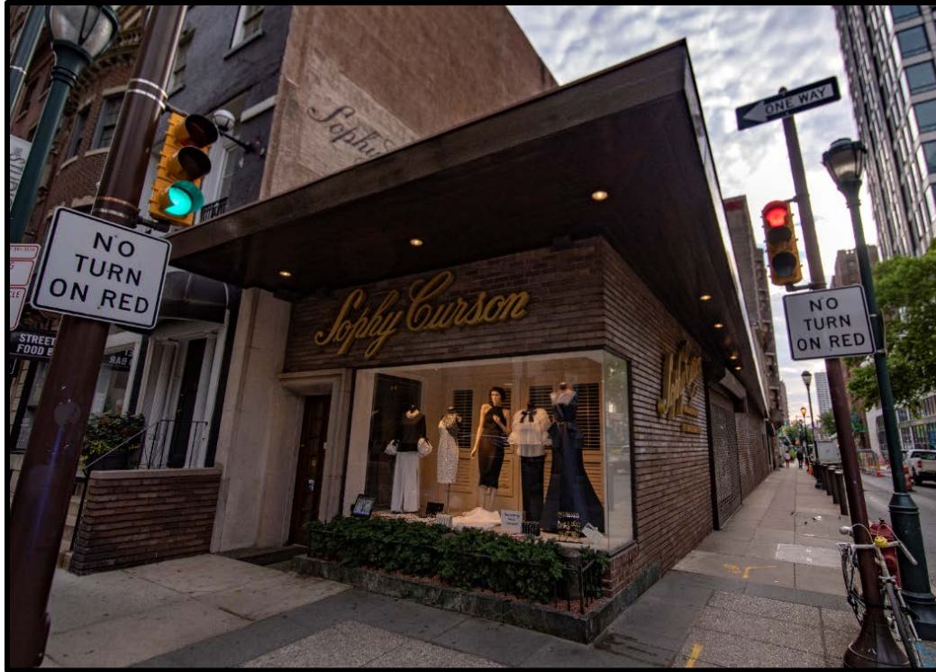
Figure 3. The east elevation of Sophy Curson, showing the original doorway and shopfront. Source: Brad Maule, 2019.
