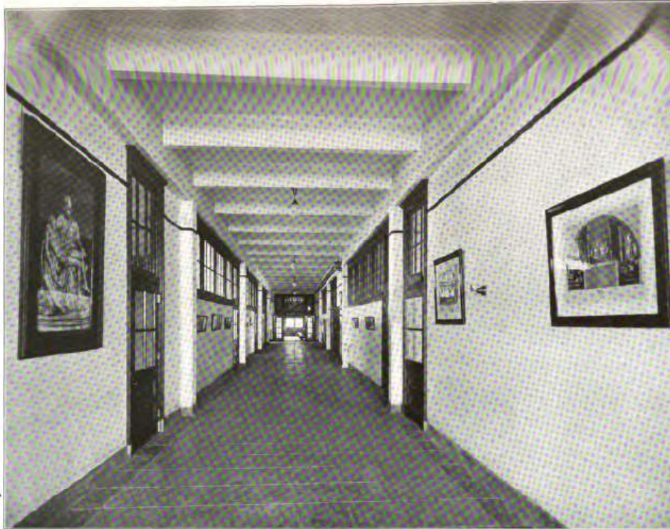
CORRIDOR CATHOLIC GIRLS' HIGH SCHOOL PHILADELPHIA CEMENT FLOOR AND BASEBOARD WITH ROUNDED ANGLES FOR THOROUGH AND EASY CLEANING
