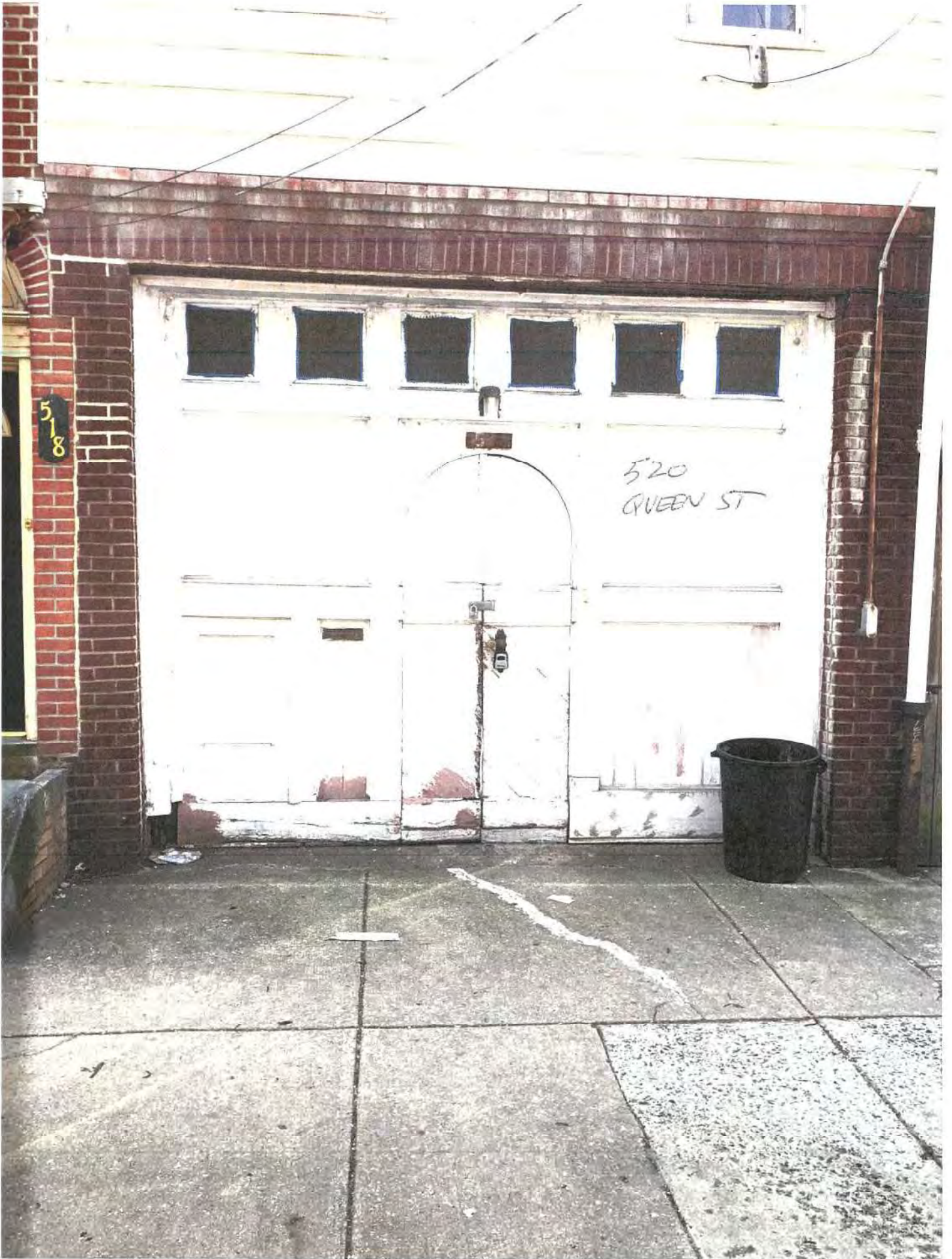
PRIMARY FRONT FACADE
