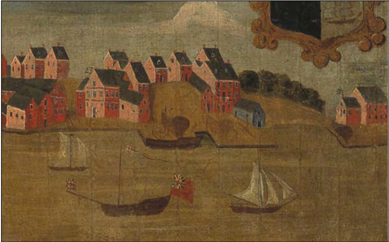
Figure 3.1. A vessel under construction at the West Shipyard (right edge of frame) with the Penny Pot house (#24) behind. Extract from The South East Prospect of the City of Philadelphia by Peter Cooper, circa 1718 (Cooper 1720).
