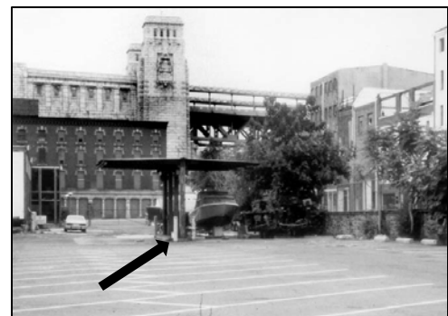
Photo 5.10. A view looking south toward Vine Street during the 1987 excavation, showing covered structure with bollards (Weber and Yamin 1988/2006, 13).
