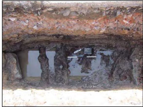
Photo 3.3. Logs forming part of a grillage wharf (Feature 6) located 6 feet below the surface of the parking lot (John Milner Associates, Inc. 2013, 32).
