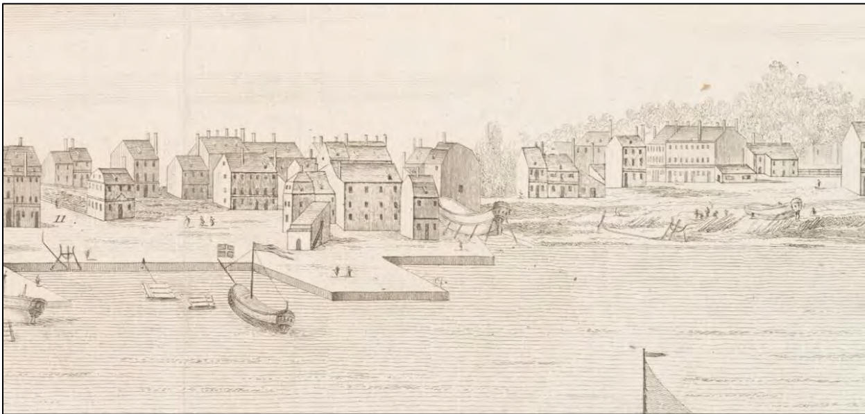
Figure 3.2. A view of the West Shipyard wharf and shipbuilding within the project area, circa 1754. Extract from An East Prospect of the City of Philadelphia by George Heap and engraved by Thomas Jeffreys (Heap, Scull and Jefferys 1754).
