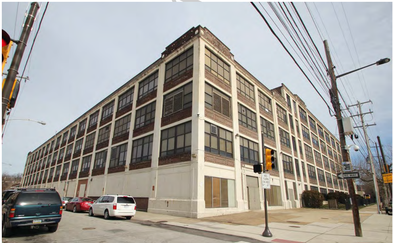
Photograph #4 – South elevation, Sections A and C, view northeast
