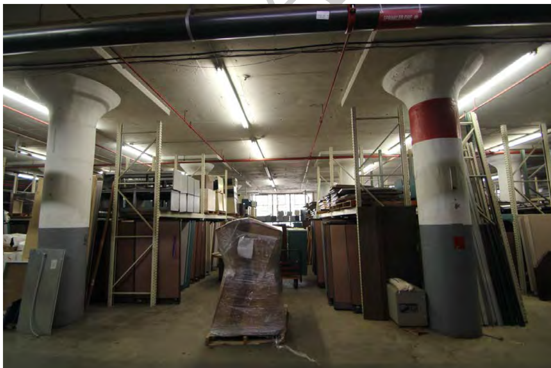
Photograph #16 – Section A, 1st floor, view west
