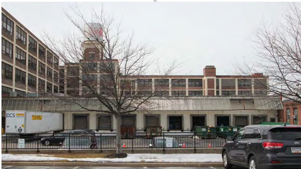
Photograph #12 – East and north elevations, Sections A, F and G, view west
