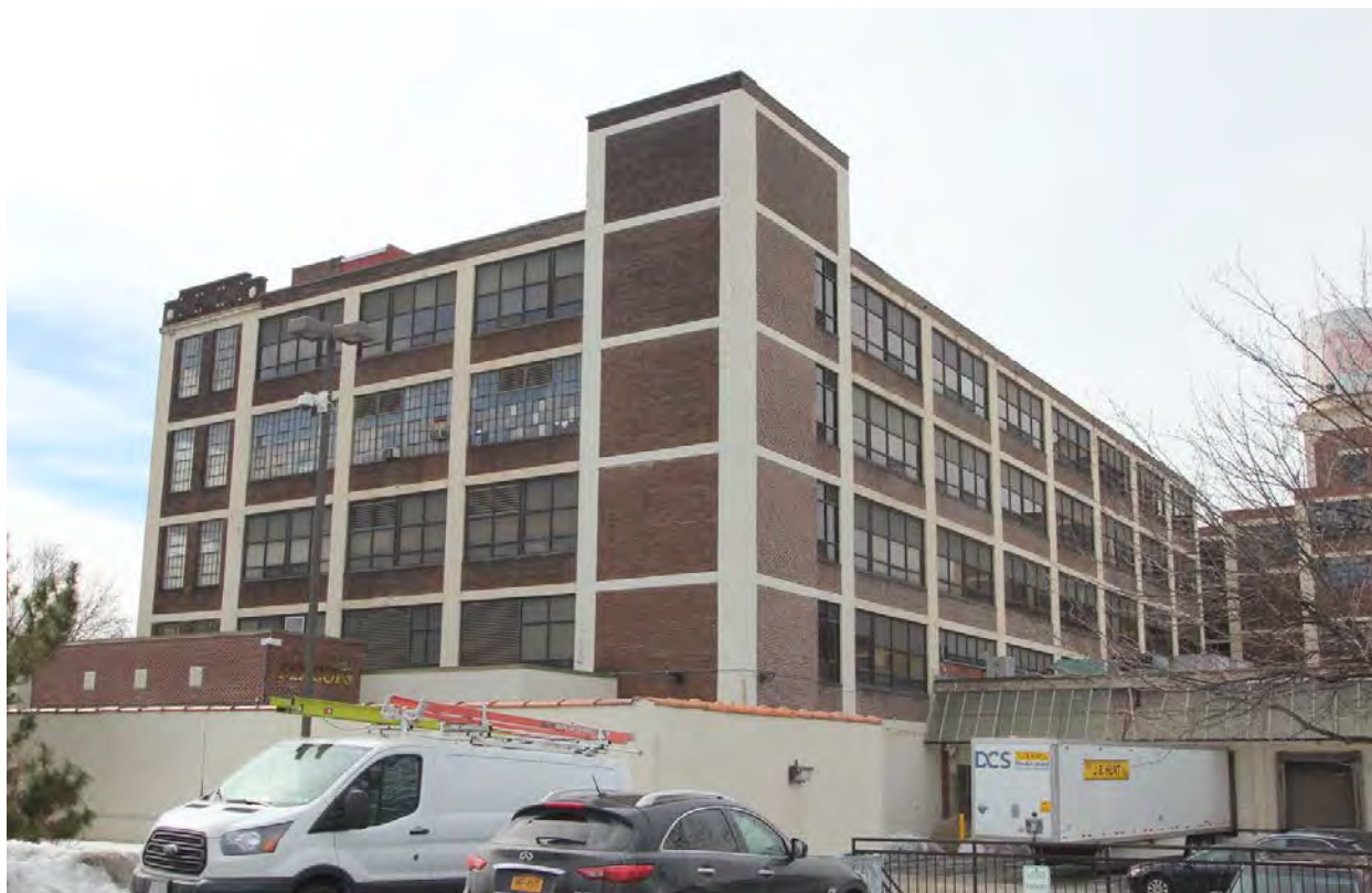
Photograph #11 – East and north elevations, Sections F, G and L, view southwest
