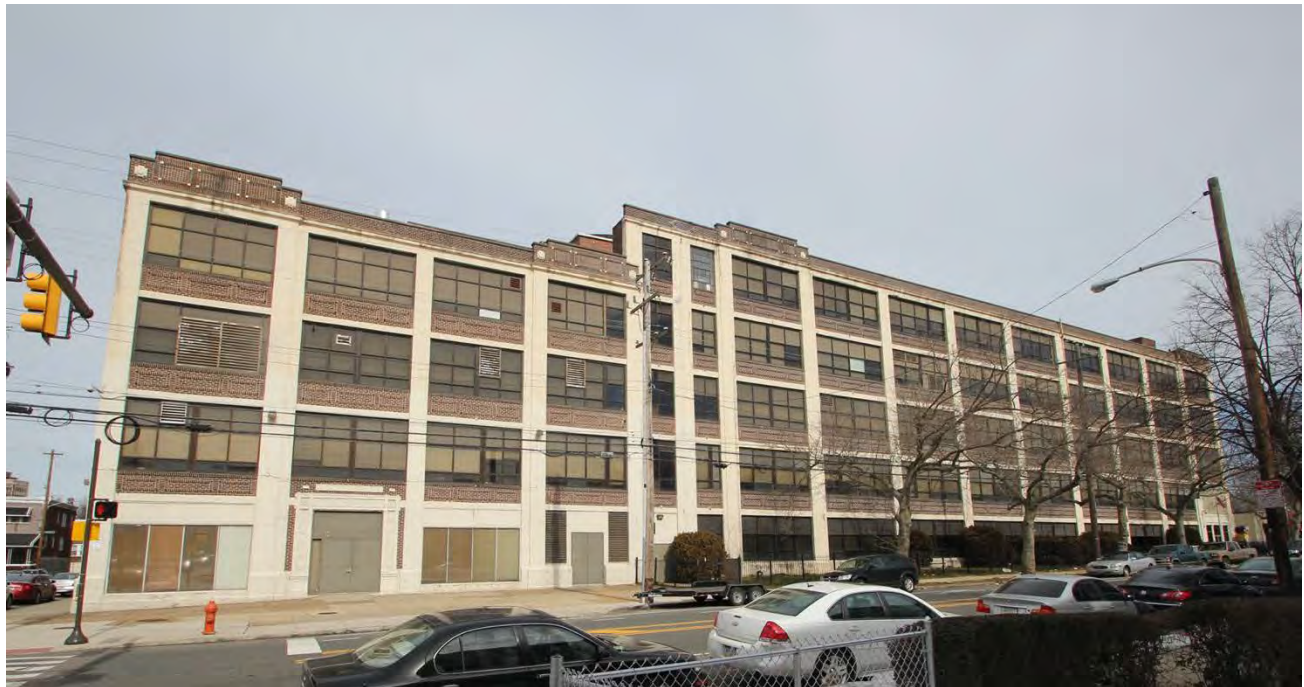
Photograph #3 – South elevation, Sections A and C, view northeast
