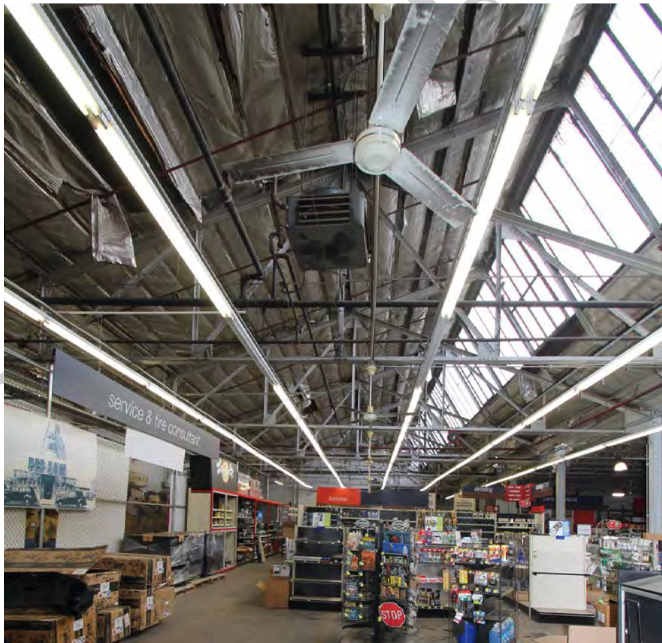
Photograph #18 – Section B, 1st floor, view west
