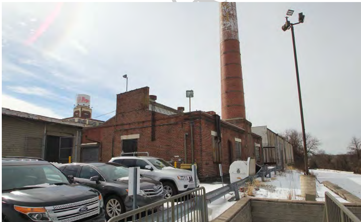
Photograph #8 – East and north elevations, Sections D, E, H and J, view SW
