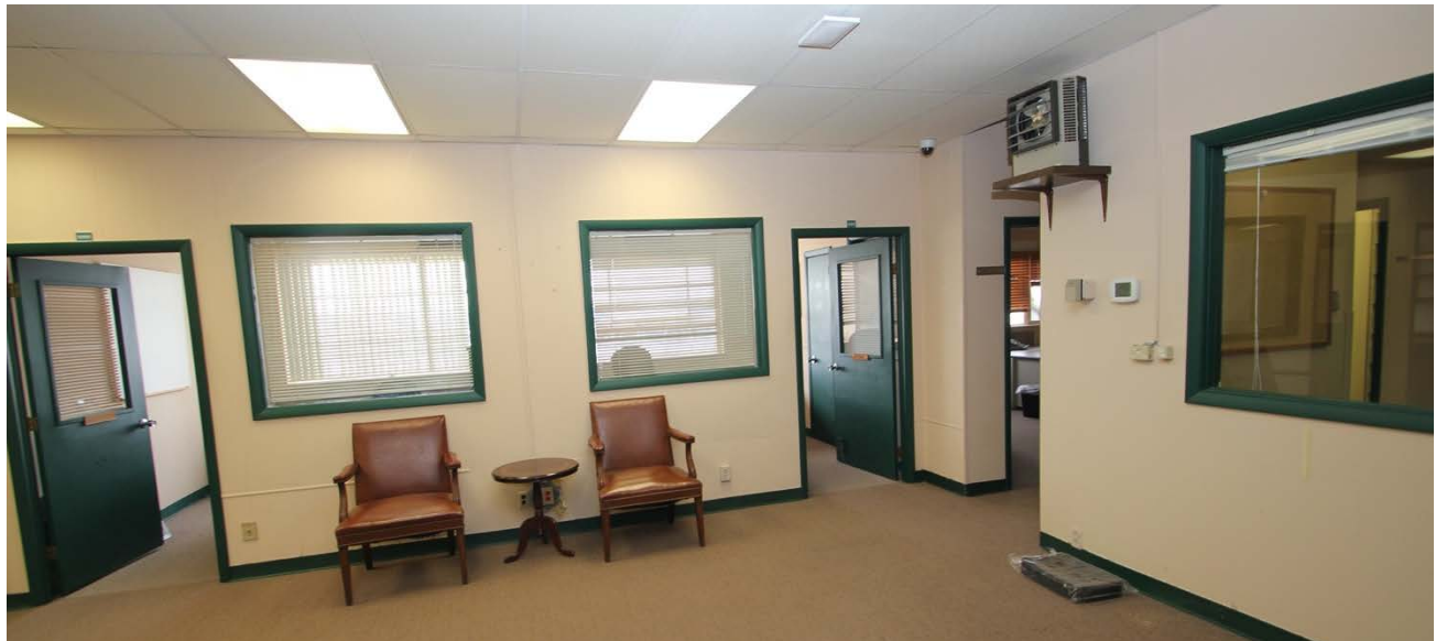
Photograph #33 – Section A, 5th floor, view west
