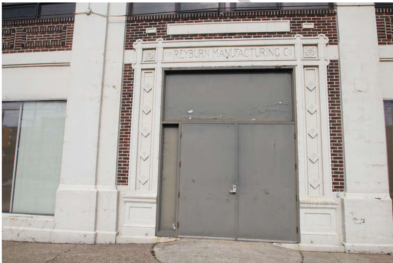
Photograph #6 – South elevation, Section A, Entrance, view north. Original entrance to the building.
