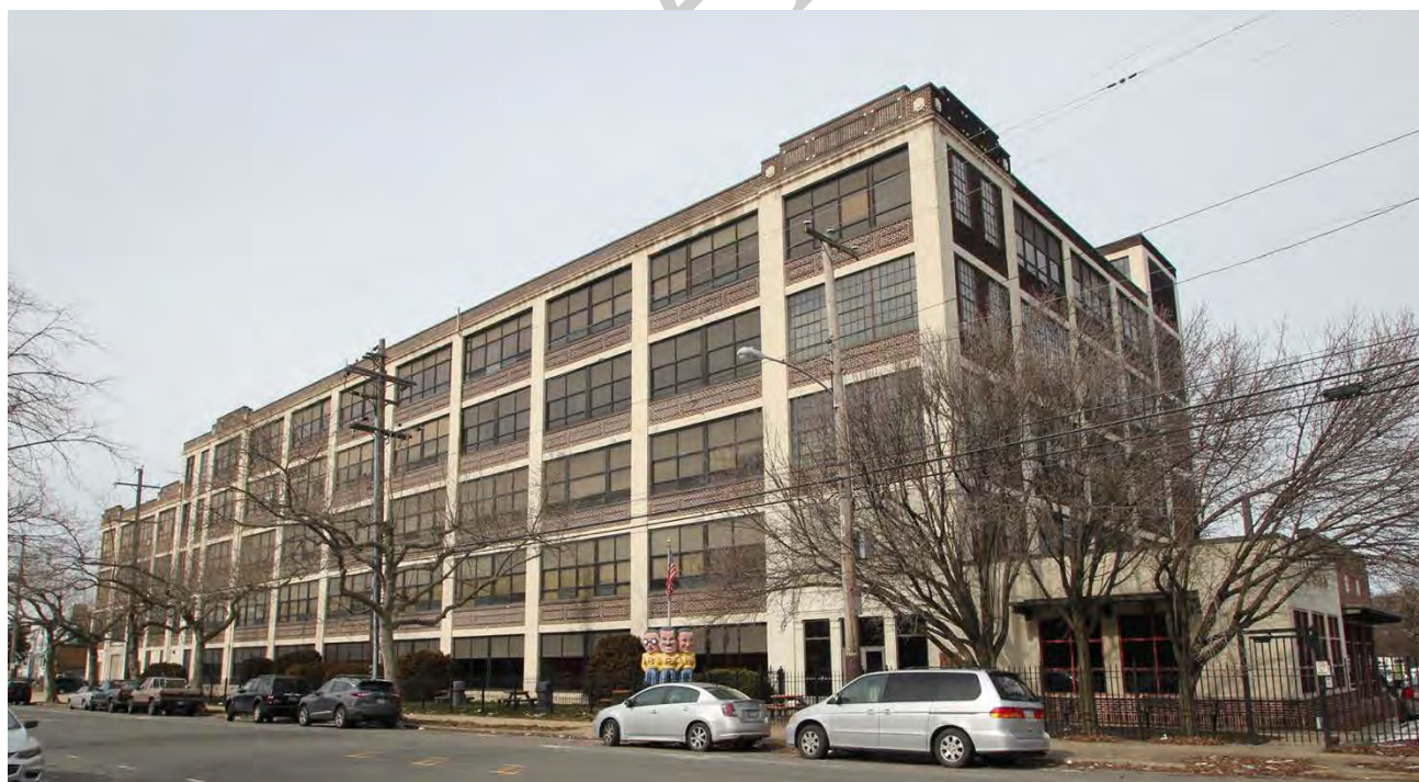
Photograph #10 – South and east elevations, Sections A, F and L, view northwest
