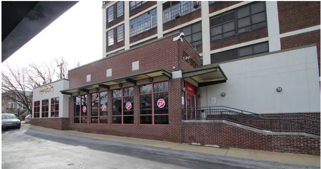
Photograph #13 – East and north elevations, Sections F and L, view southwest. Section L was constructed outside of the Period of Significance.
