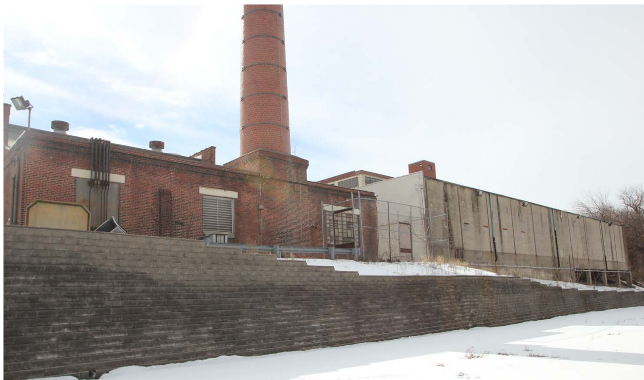
Photograph #9 – East and north elevations, Sections D, E and H, view southwest
