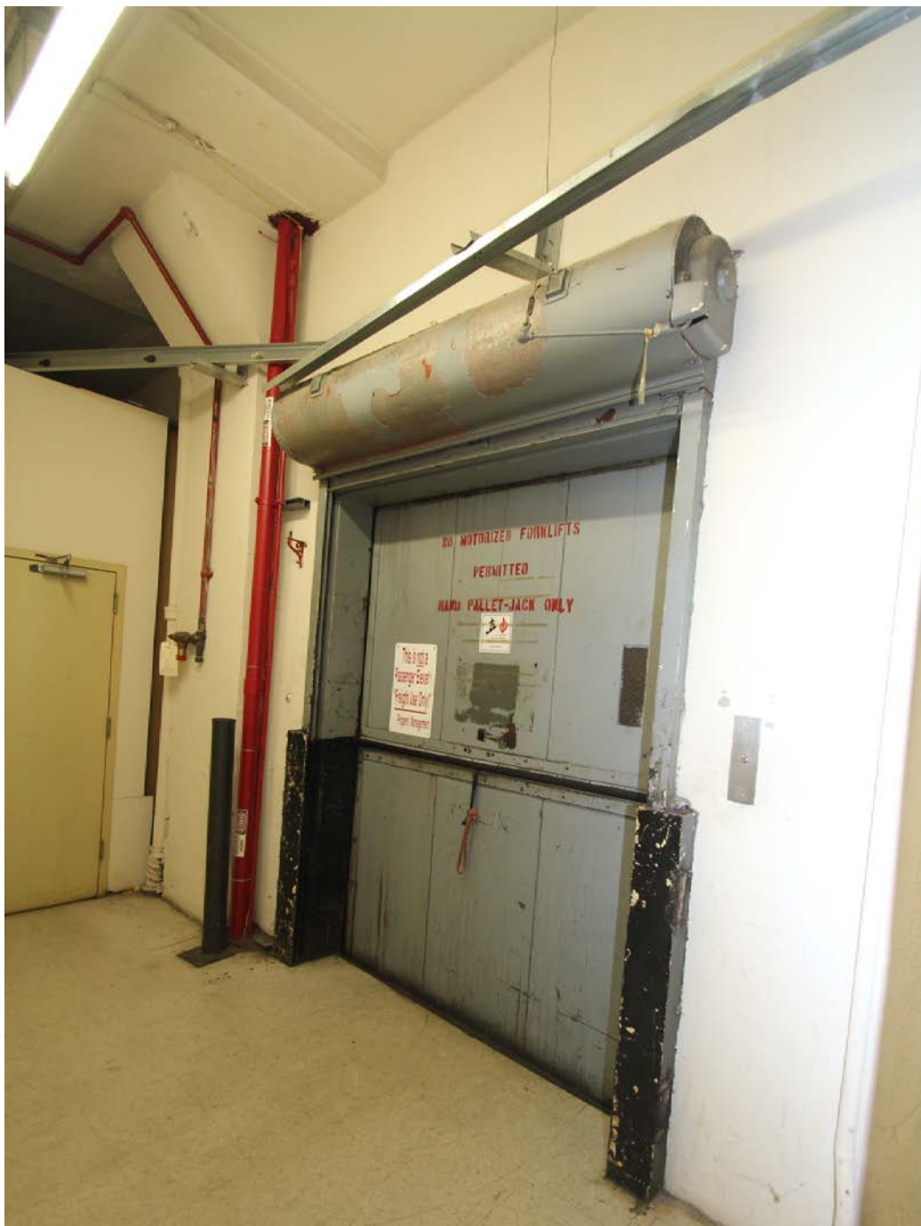
Photograph #36 – Section A, 2nd floor, Elevator, view northeast
