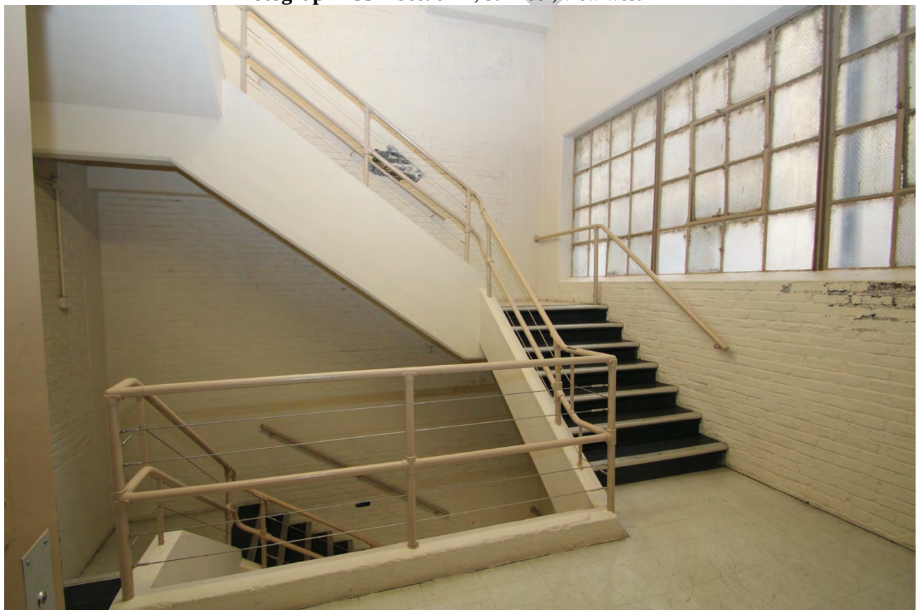
Photograph #34 – Section A, 2nd floor, Stairway, view east
