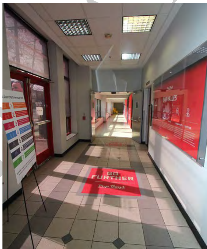
Photograph #20 – Section F, 1st floor, view west
