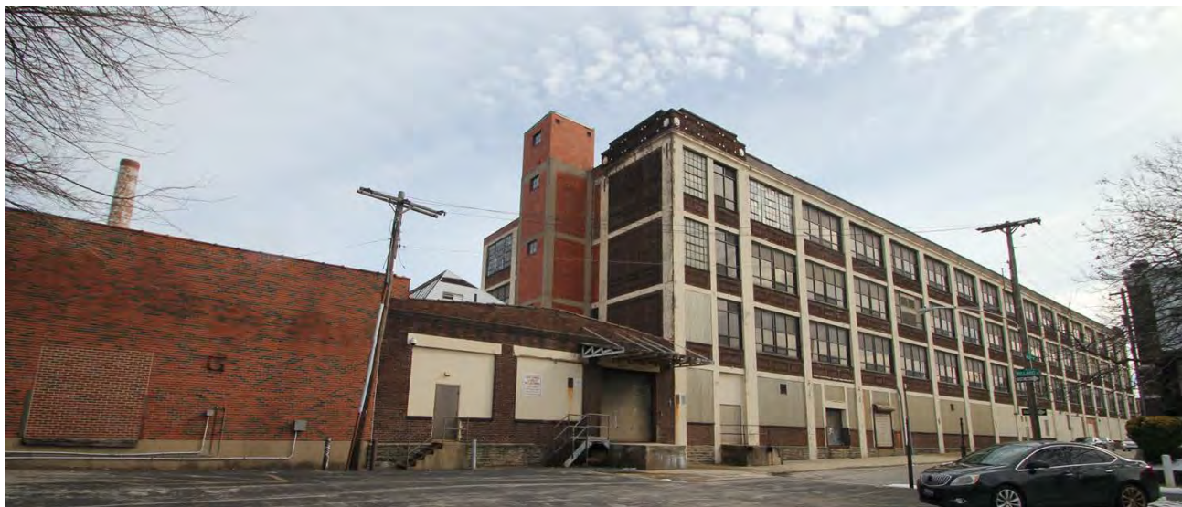
Photograph #5 – West and north elevations, Sections A, B and H, view southeast
