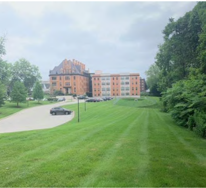
VIEW FROM CENTER LACONIA TO NUGENT BUILDING ▲
