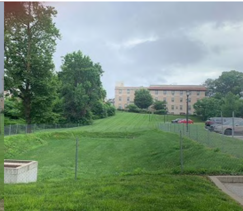
VIEW FROM CENTER LACONIA TO PRESSER BUILDING ▲
