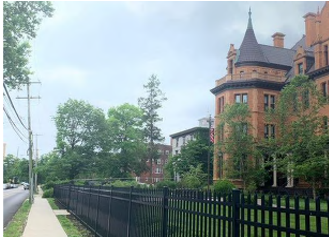
VIEW FROM WEST JOHNSON TO ARDS NUGENT BUILDING ▲
