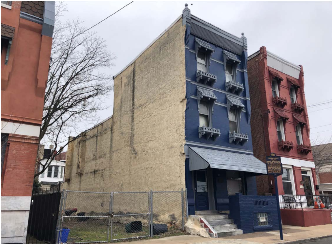
Figure 7: Stuccoed south elevation party wall and east front elevation. March 2021. Philadelphia Historical Commission staff.
