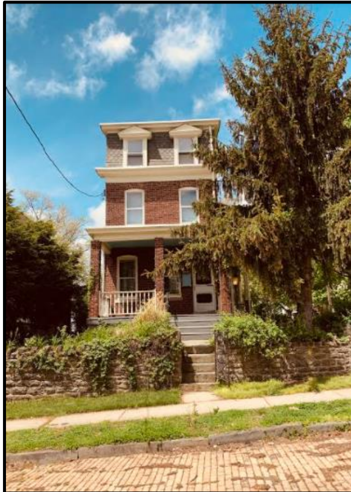
Figure 1. The primary (southeast) elevation of the subject property. Source: Oscar Beisert.
