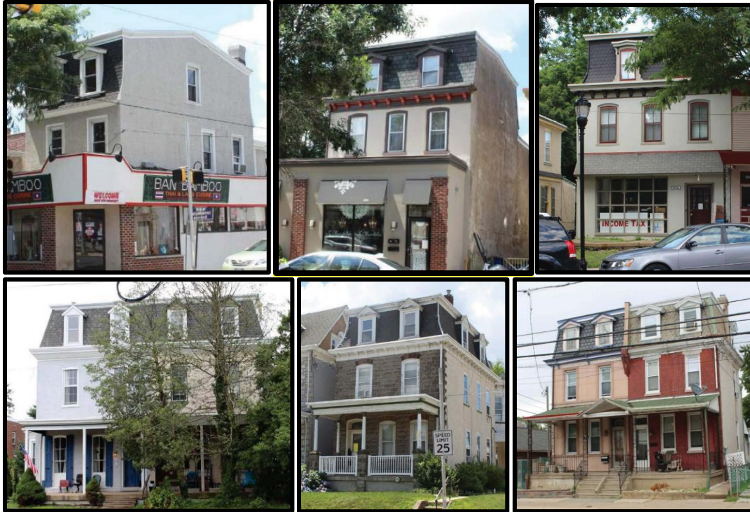
Examples of the Second Empire style in the domestic architecture of Ridge Avenue and Roxborough. Figure 26. Top left: 6190 Ridge Avenue (ca.1875-84). Figure 27. Top center: 6212 Ridge Avenue (ca.1886-88). Figure 28. Top right: 6234 Ridge Avenue (ca.1883-84). Figure 29. Bottom left: 7910 and 7912 Ridge Avenue (ca.1875-84) Figure 30. Bottom center: 6526 Ridge Avenue (ca.1900). Figure 31. Bottom right: 6787 and 6789 Ridge Avenue (ca.1900). Source: Philadelphia Register of Historic Places Nomination: Ridge Avenue Roxborough Thematic Historic District.
