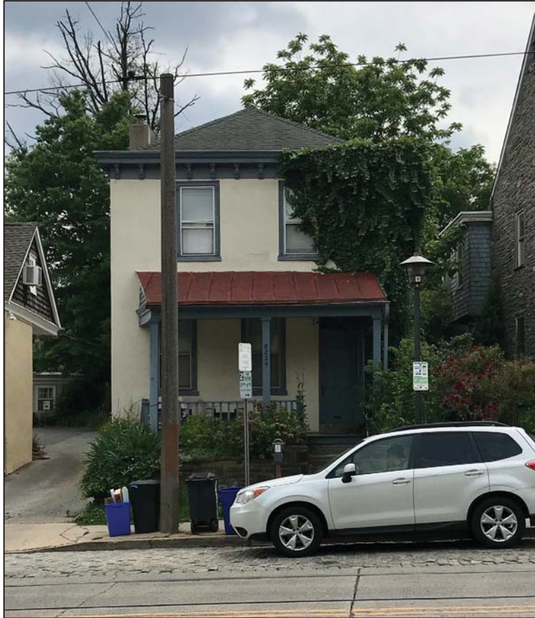
Fig. 6. The primary elevation of the dwelling showing the hipped roof, front porch construction, two bay upper floor and front door to the north of two ground floor windows, all elevated above sidewalk and street level with shared driveway with building to the south.
