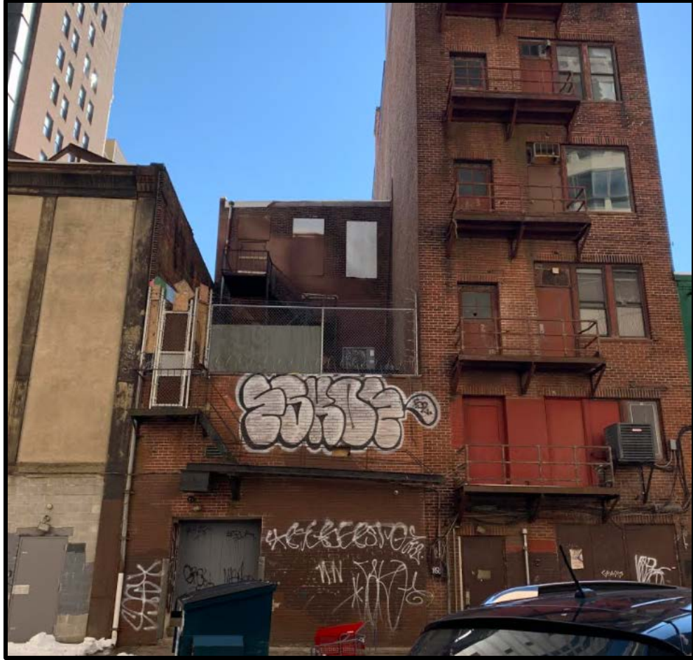
Figure 7. Looking south at the rear (north) elevation. Source: Oscar Beisert, 2021.
