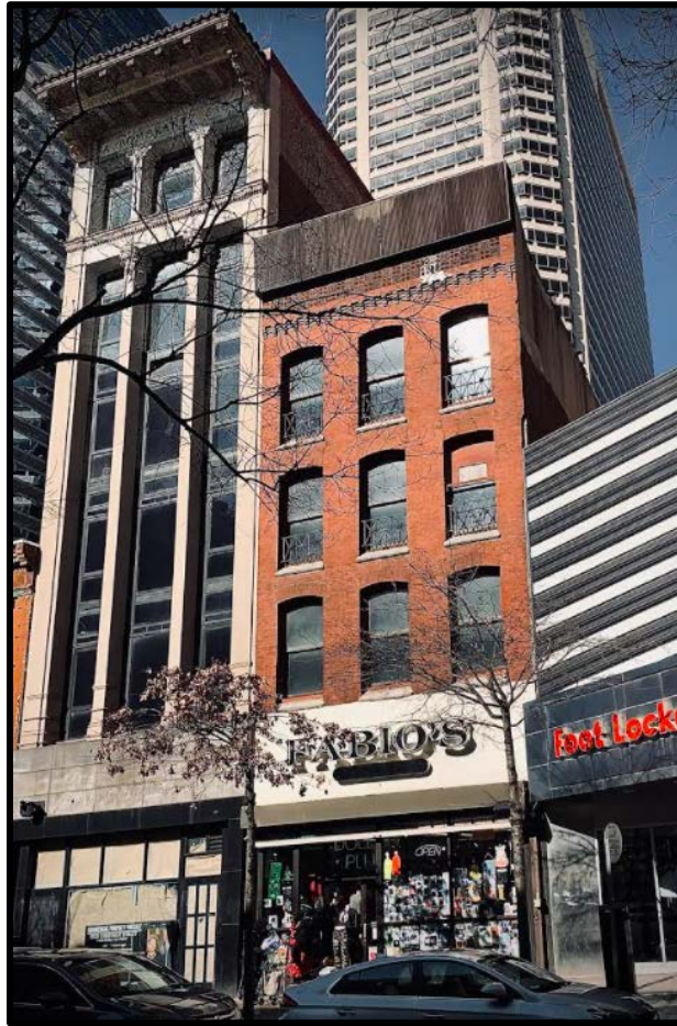
Figure 1. The primary (south) elevation. Source: Oscar Beisert, 2021.
