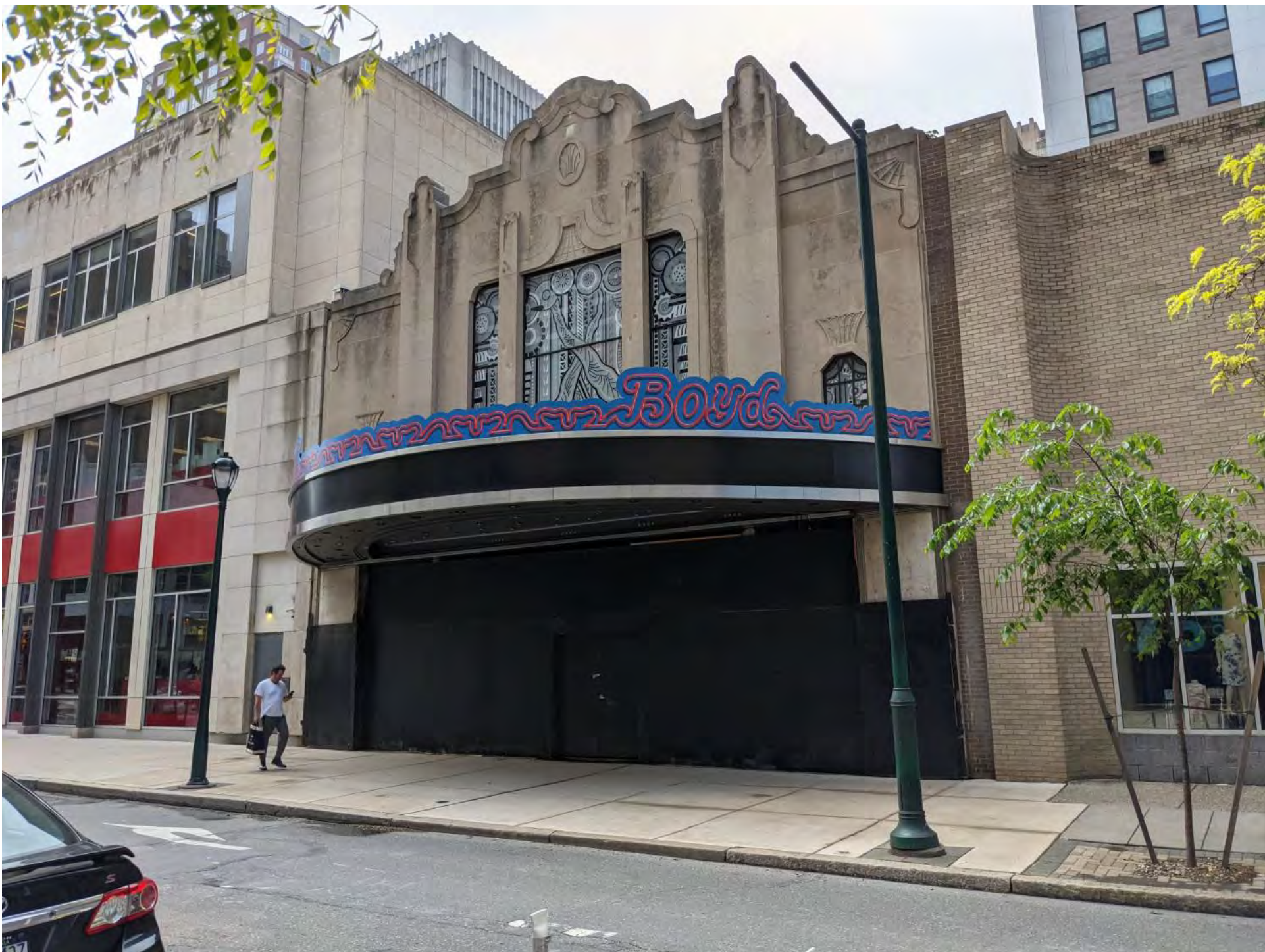
EXISTING MARQUEE TO REMAIN AND BE RESTORED. NEW ILLUMINATED CHANNEL LETTERING TO OCCUPY 2'-0" BLACK BAND
