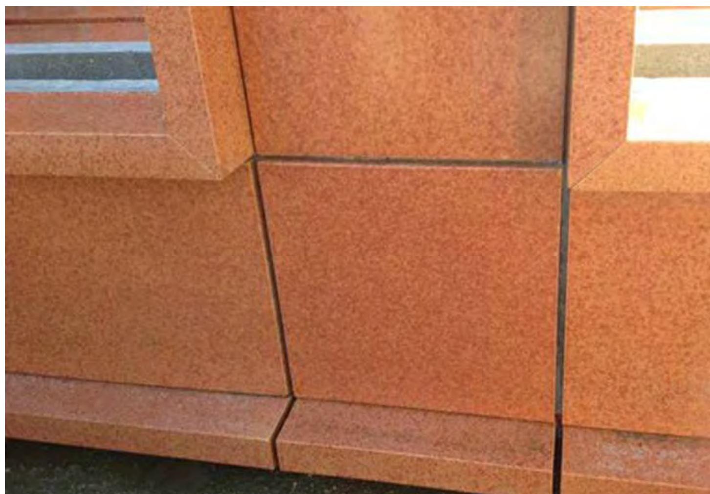
BOSTON VALLEY TERRA COTTA PRE-CAST PANELS, SLATE COLOR
