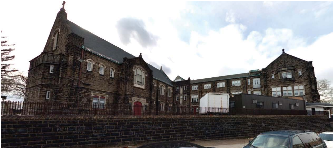
Figure 7: Northeast elevation of chapel and southeast elevation of northeastern wing, from N. 29 th Street.
