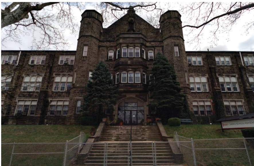
Figure 3: Detail of primary entrance on W. Hunting Park Avenue.
