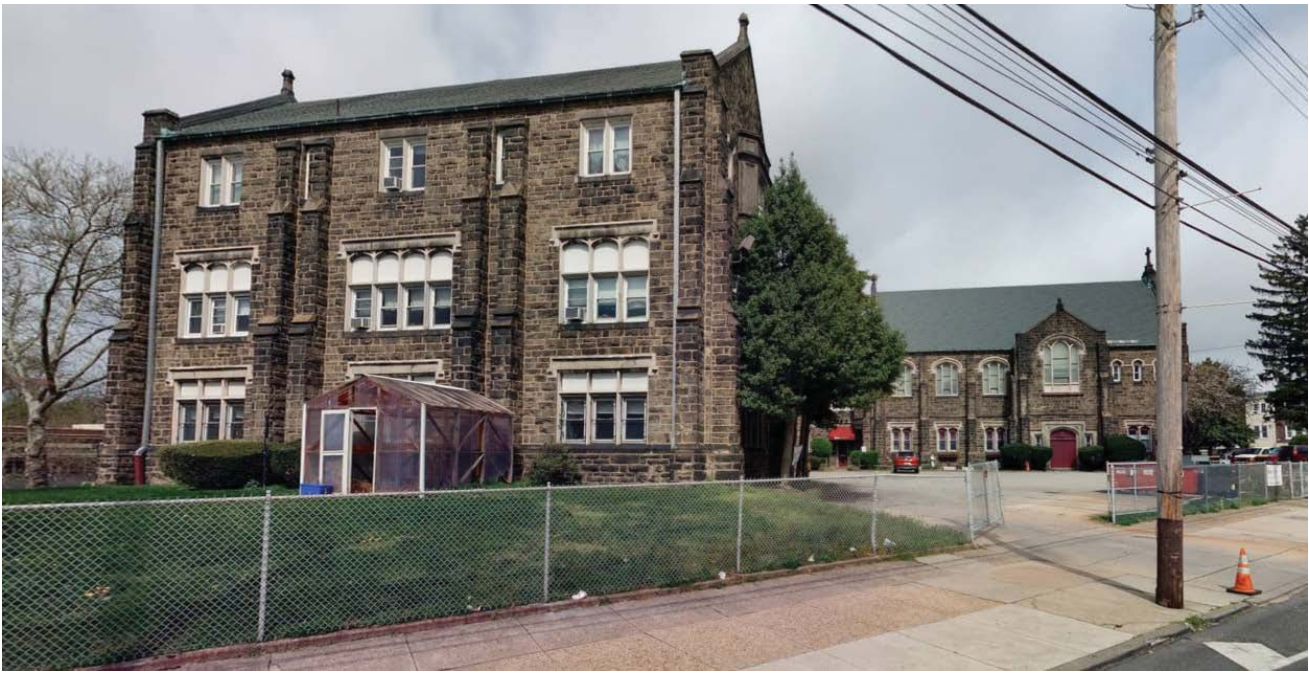
Figure 4: Southwest elevation of southwestern wing, with southwest elevation of chapel in background, from W. Allegheny Avenue.
