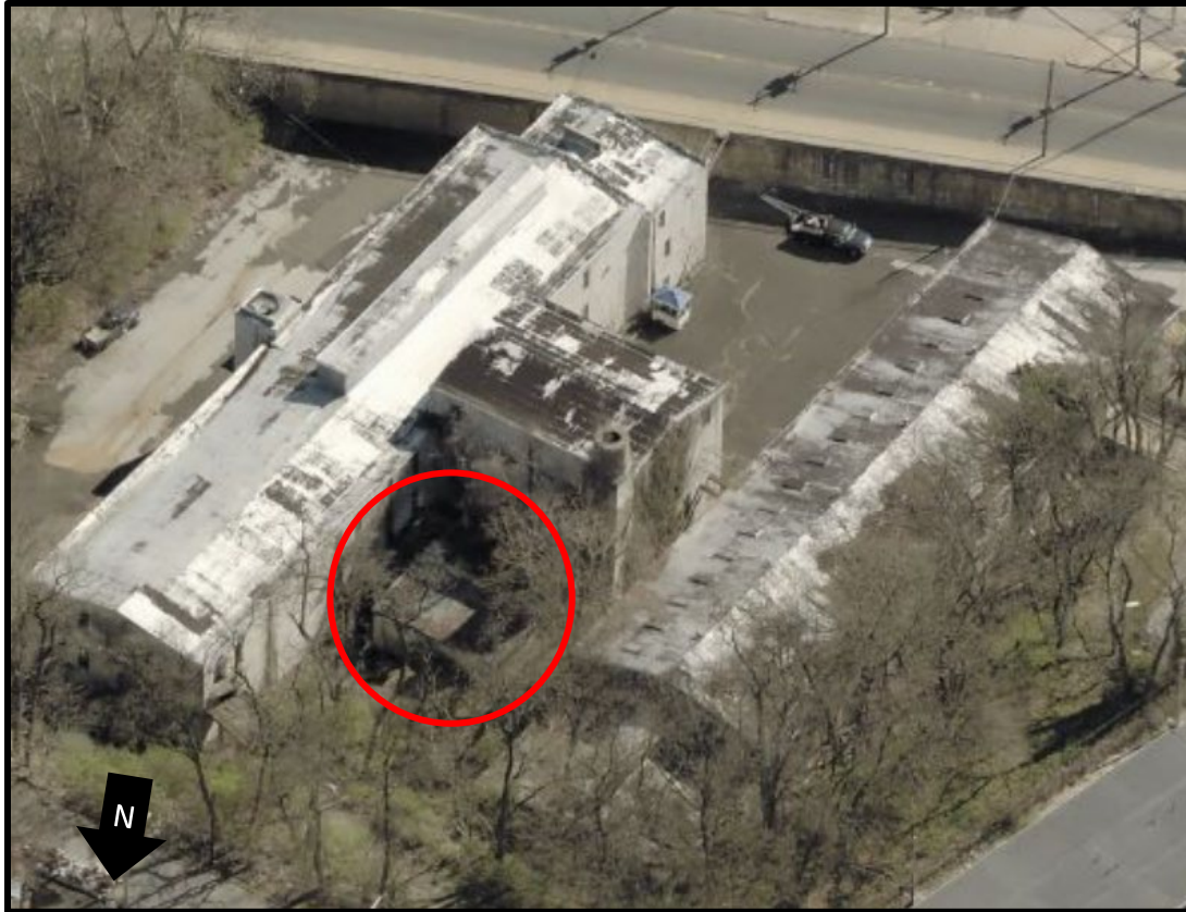
Figure 27. Looking south, a bird's eye view of the subject property with the rear (north) and side (west) elevations of Building 9 circled. Source: Pictometry, Atlas, City of Philadelphia.
