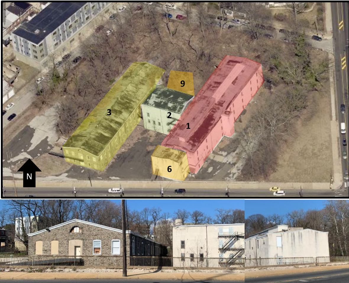
Figure 4. Top: Looking north from a bird’s eye view of the subject property showing all of the extant buildings, as labeled based on historic atlases. Source: Pictometry, Atlas, City of Philadelphia. Figure 5. Bottom: Looking north at the subject property. Source: Oscar Beisert, 2020.
