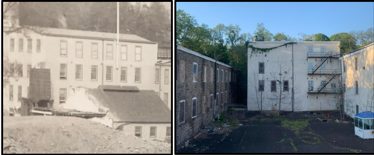
Figure 16. Left: Looking northeast at Building 2 in 1902. Source: The Philadelphia Gas Works Photograph Collection, City Archives of Philadelphia. Figure 17. Right: The primary (south) elevation of Building 2. Source: Oscar Beisert, 2020.
