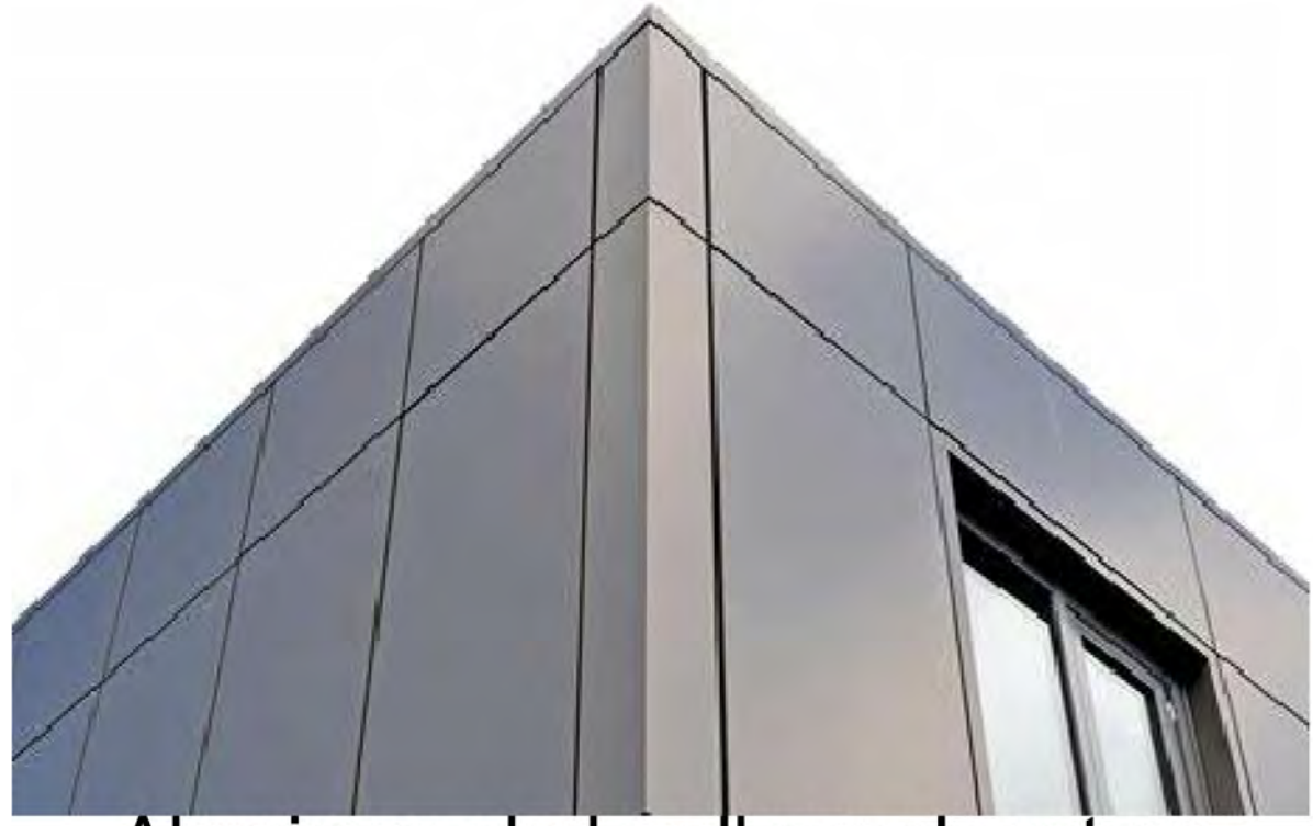
Aluminum clad wall panel system 3 Grey tones Blue accent Bands
