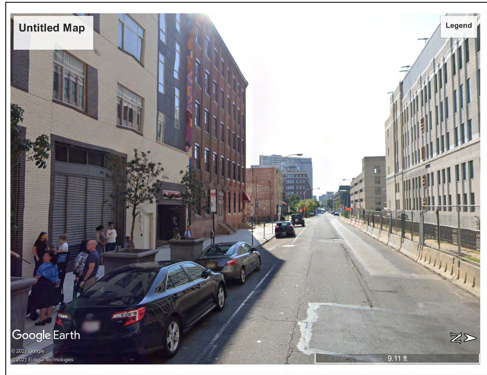
IMAGE 4 VIEW, CALLOWHILL WEST TO 15TH ST. PARKING ENTRANCE TO BUILDINGS AND LOUVERED WALLS FOR MECHANICAL SYSTEM ADORN STREETSCAPE
