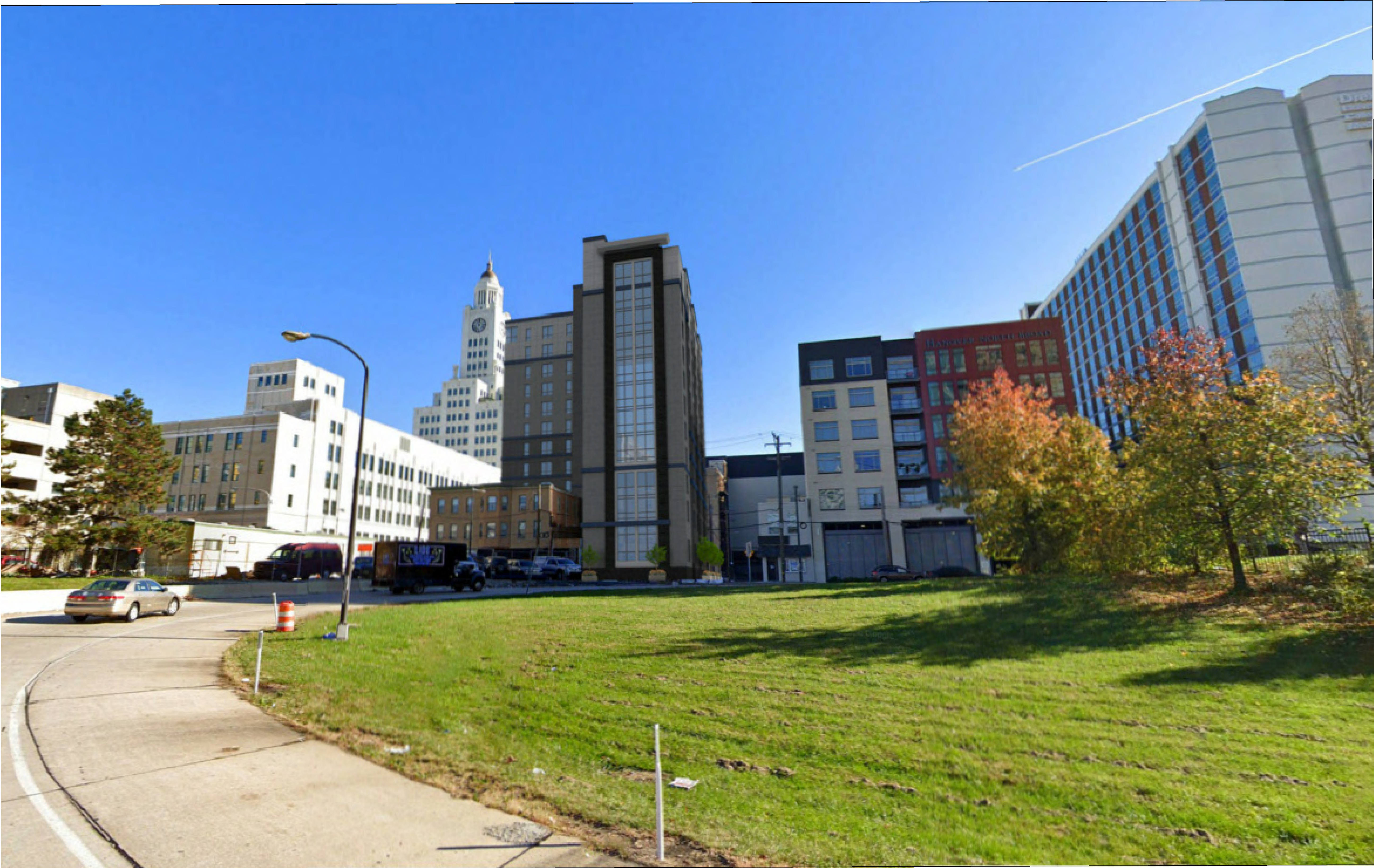
THE 15 ST ST SIDE OF THE SITE IS VIEWED FROM ONE OF THE MAJOR ENTRY POINTS TO CC. THE 15TH ST CORRIDOR IS HOME TO MANY BUILDINGS WITH VERTICAL MASSING, AS WELL AS THE VISIBLE TOWER IN THE UPPER LEFT. THIS SITE HAS THE OPPORTUNITY TO EXPRESS THOSE PROPORTIONS CARRYING ON A TRADITION OF THIS URBANISM AS ESTABLISHED BY THE TOWER TO THE LEFT AND THE 1960'S STRUCTURE TO THE RIGHT
