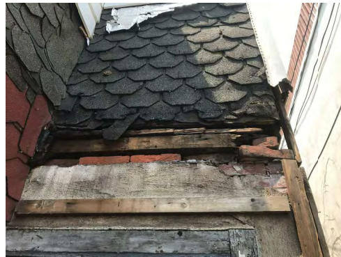
DETERIORATED CONDITIONS UNDER SIDING
