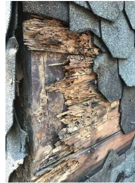
DETERIORATED CONDITIONS UNDER SIDING
