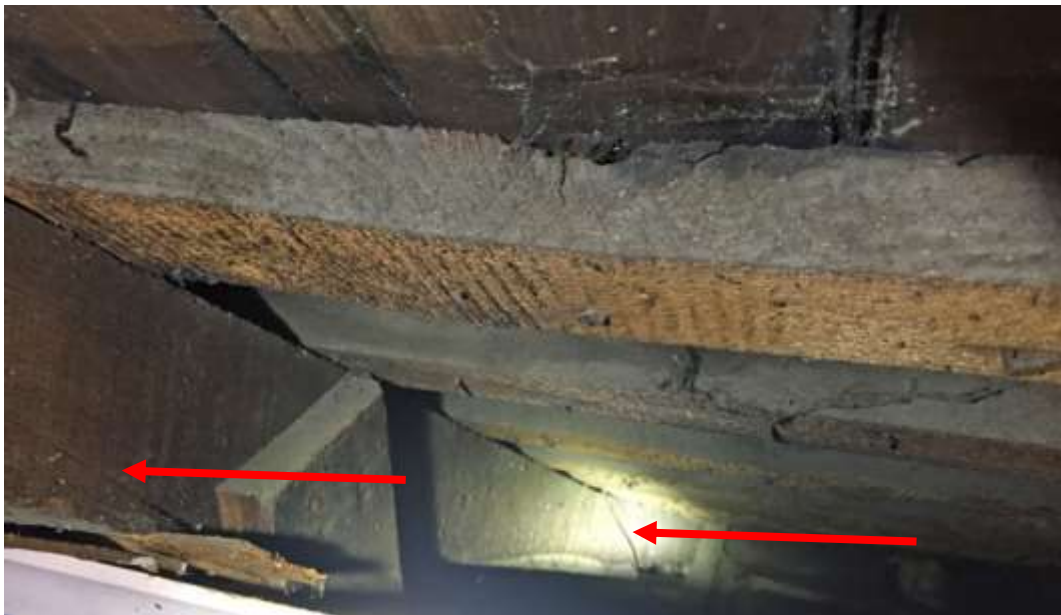
Cracks entirely through undersized roof rafter. Every rafter inspected had similar problems.
