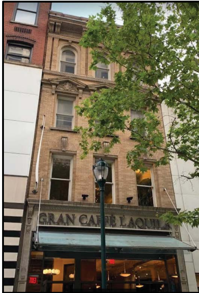
Figure 1. The primary (north) elevation of the Wall & Ochs Building. Source: Oscar Beisert, 2020.
