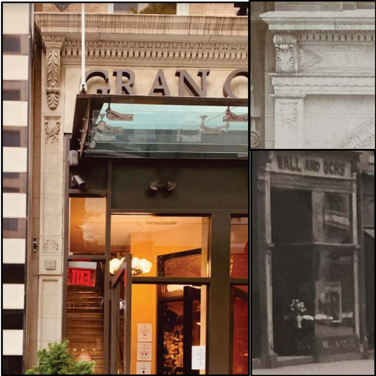
Figure 4. Left: A detail of the current terra cotta storefront surround of the primary (north) elevation. Source: Oscar Beisert, 2020. Figure 5. Top right: An early photograph of the Wall & Ochs Building, showing a detail of the terra cotta of the first floor, suggesting that the upper portion may date to the original construction. Source: Frank Taylor Photographs, The Free Library of Philadelphia. Figure 6. Bottom right: A later photograph of the Wall & Ochs Building, showing the storefront as it was in the 1920s, the surround of which appears to be largely intact. Source: The Boies Penrose Collection, The Historical Society of Pennsylvania.
