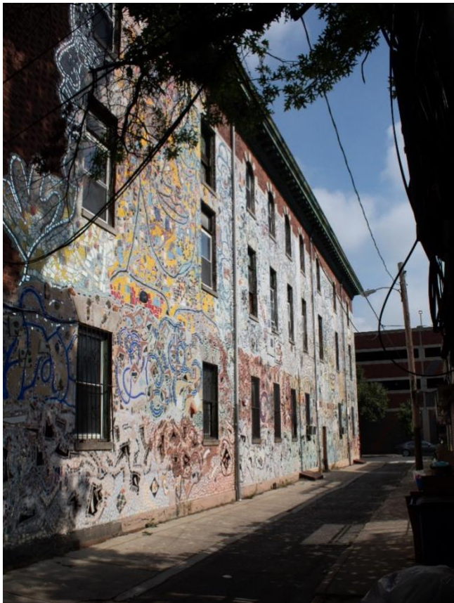
Figure 6 East elevation, 1016-18 South Street. (Source: Author, 2020)
