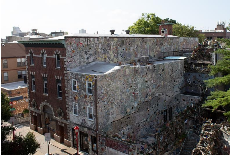
Figure 8 West elevation, 1016-18 South Street. (Source: Author, 2020)
