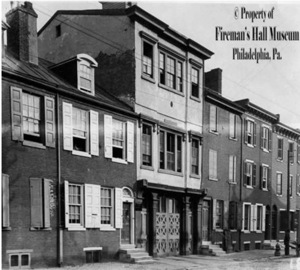
Figure 12 Engine Company 11, 1035 Lombard Street, center, c 1870s-1880s. (Source: Fireman's Hall Museum)
