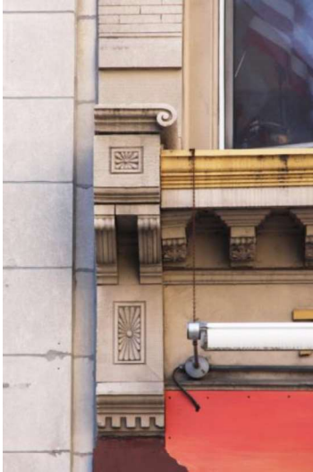
Photo 2 (left) – Detail of the limestone cornice above the first floor storefront.
