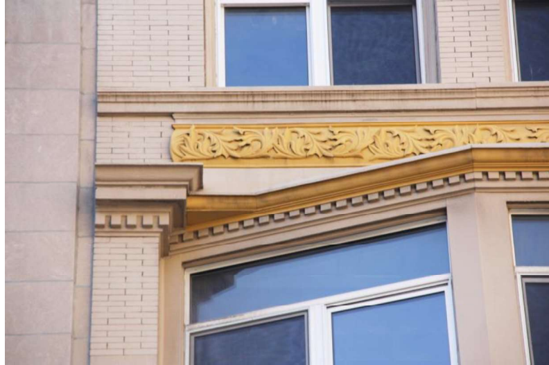
Photo 2 (left) – Detail of the limestone cornice above the first floor storefront.
