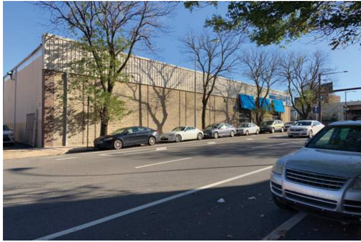
NORTHWEST CORNER OF SITE FACING SOUTHEAST
