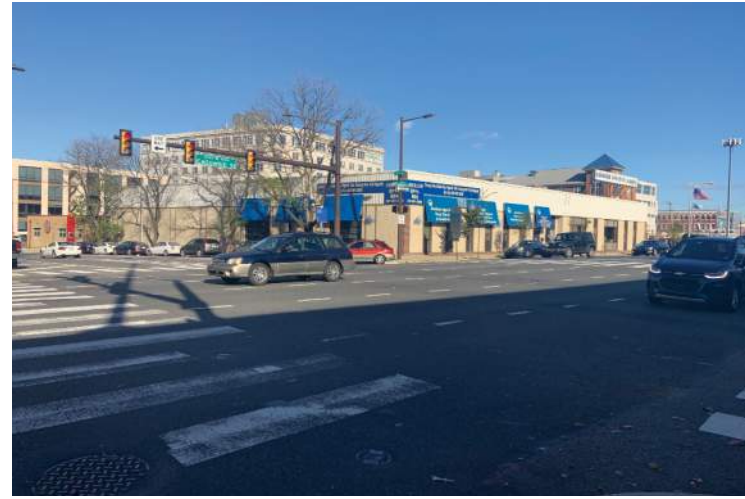
SOUTHWEST CORNER OF SITE FACING NORTH EAST
