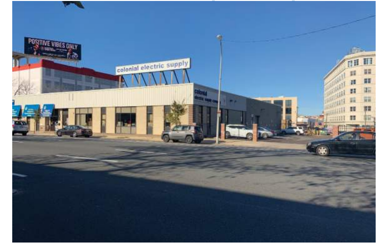
SOUTHERN EDGE OF SITE FACING NORTHWEST
