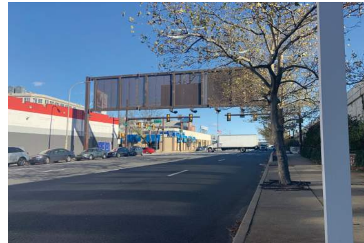
SOUTHEAST ON CALLOWHILL STREET LOOKING NORTHEAST
