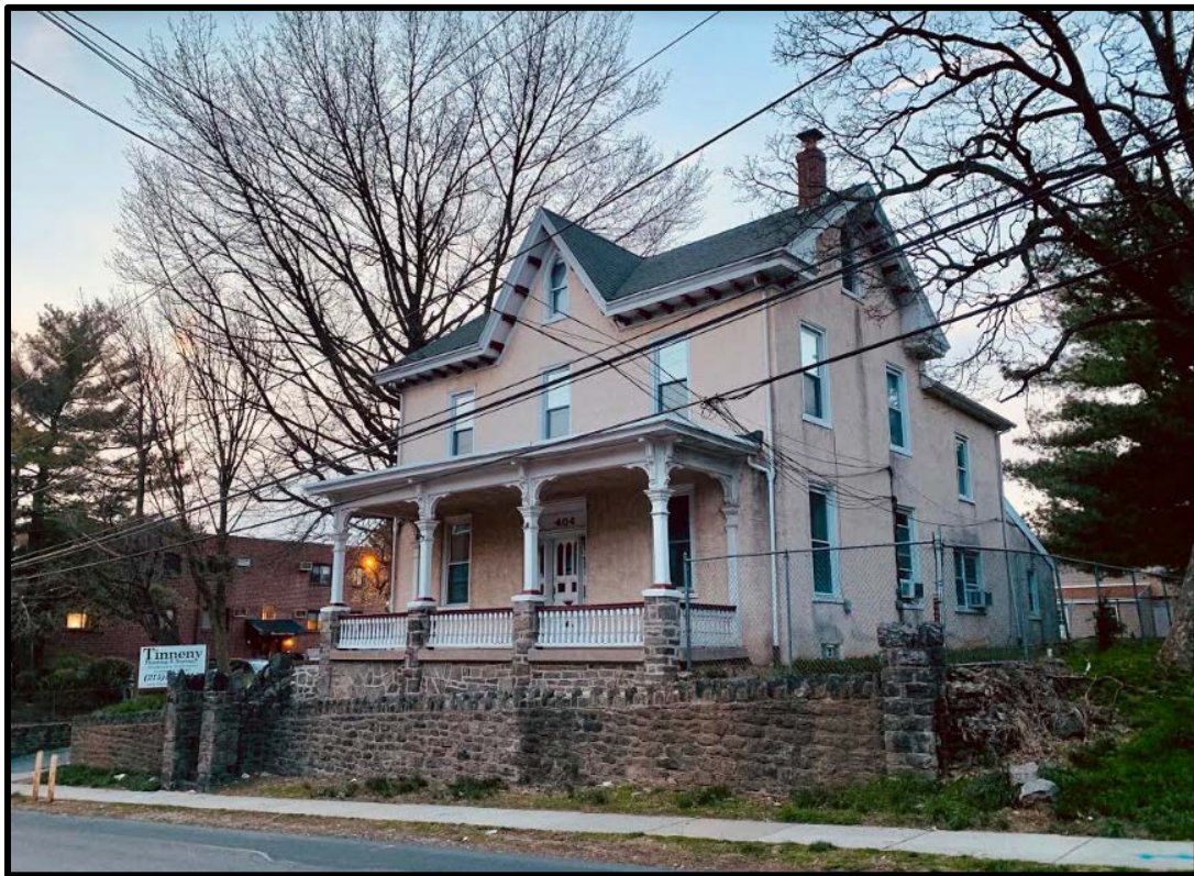
Figure 1. The primary (southeast) and side (northeast) elevations. Source: Oscar Beisert, 2021.
