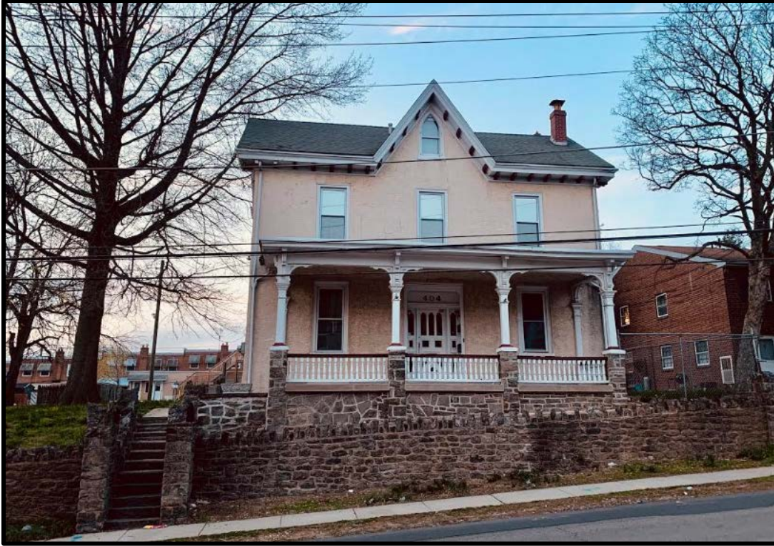
Figure 3. The primary (south) elevation. Source: Oscar Beisert, 2021.
