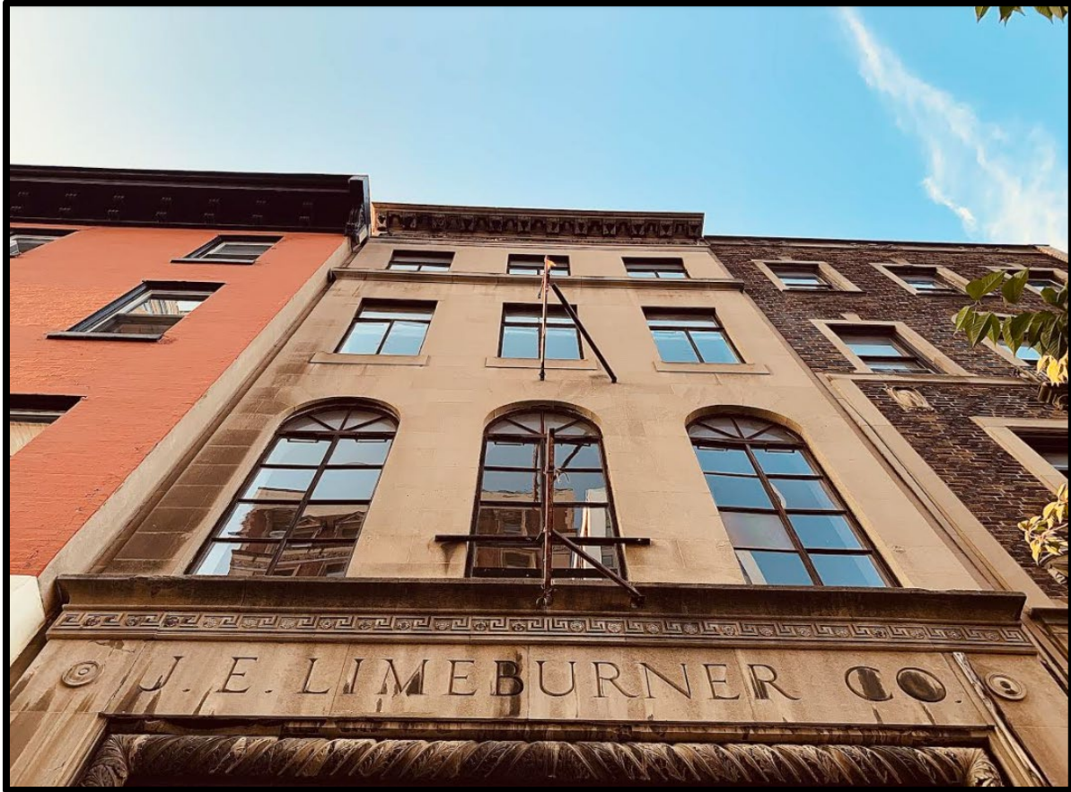
Figure 6. A view of the banner on the first floor and the upper floors of the J.E. Limeburner Co. Store. Source: Oscar Beisert, 2020.
