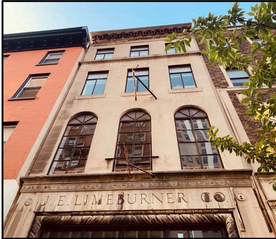
Figure 1. The primary (south) elevation of the subject property. Source: Oscar Beisert, 2020.
