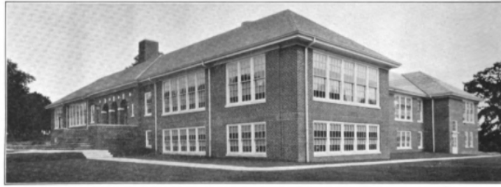
HEACOCK & HOKANSON, Architects, Philadelphia, Pa. JENKINTOWN HIGH SCHOOL, JENKINTOWN, MONTGOMERY CO., PA.
