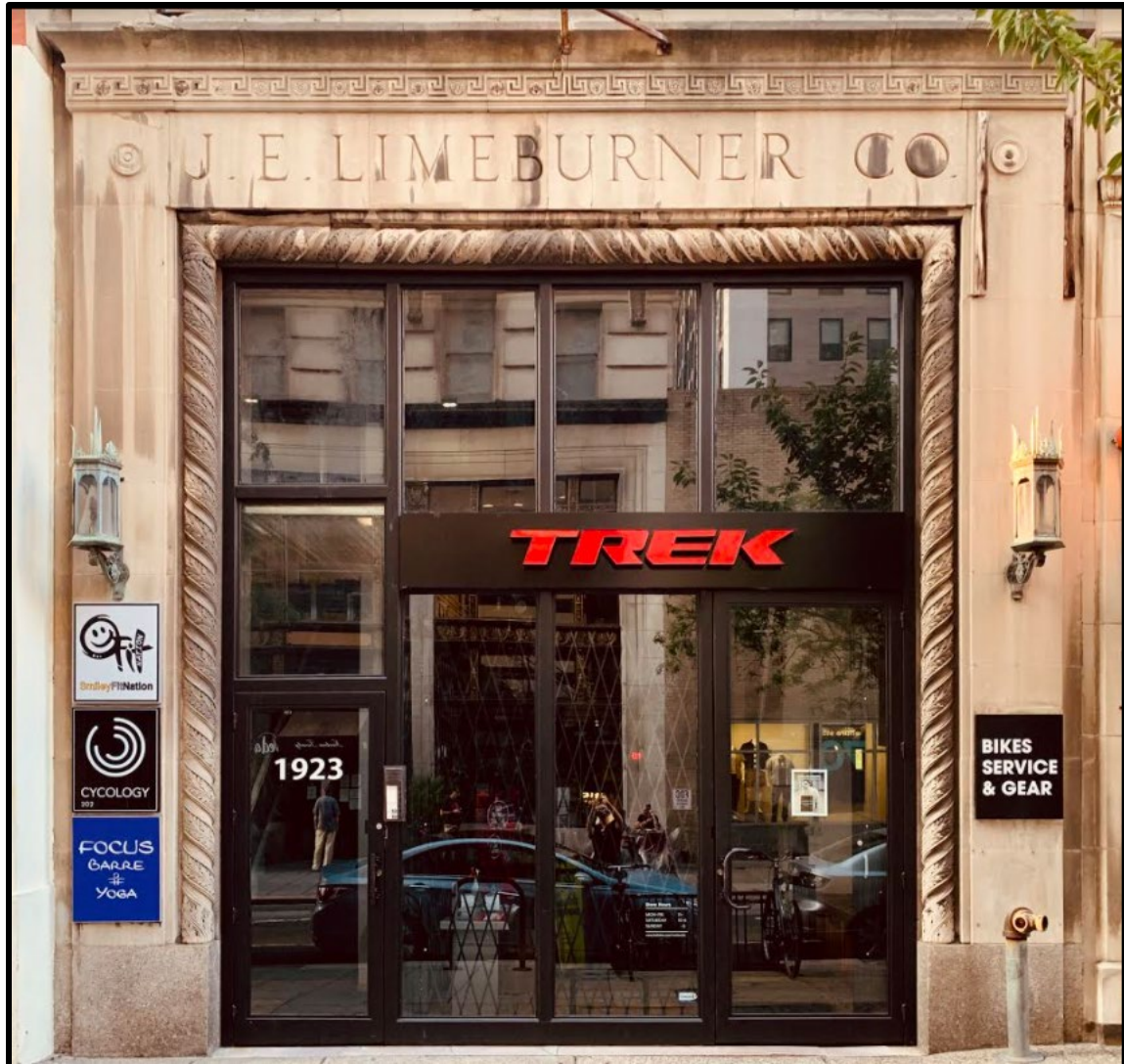
Figure 4. The primary (south) elevation of the storefront of the J.E. Limeburner Store. Source: Oscar Beisert, 2020.
