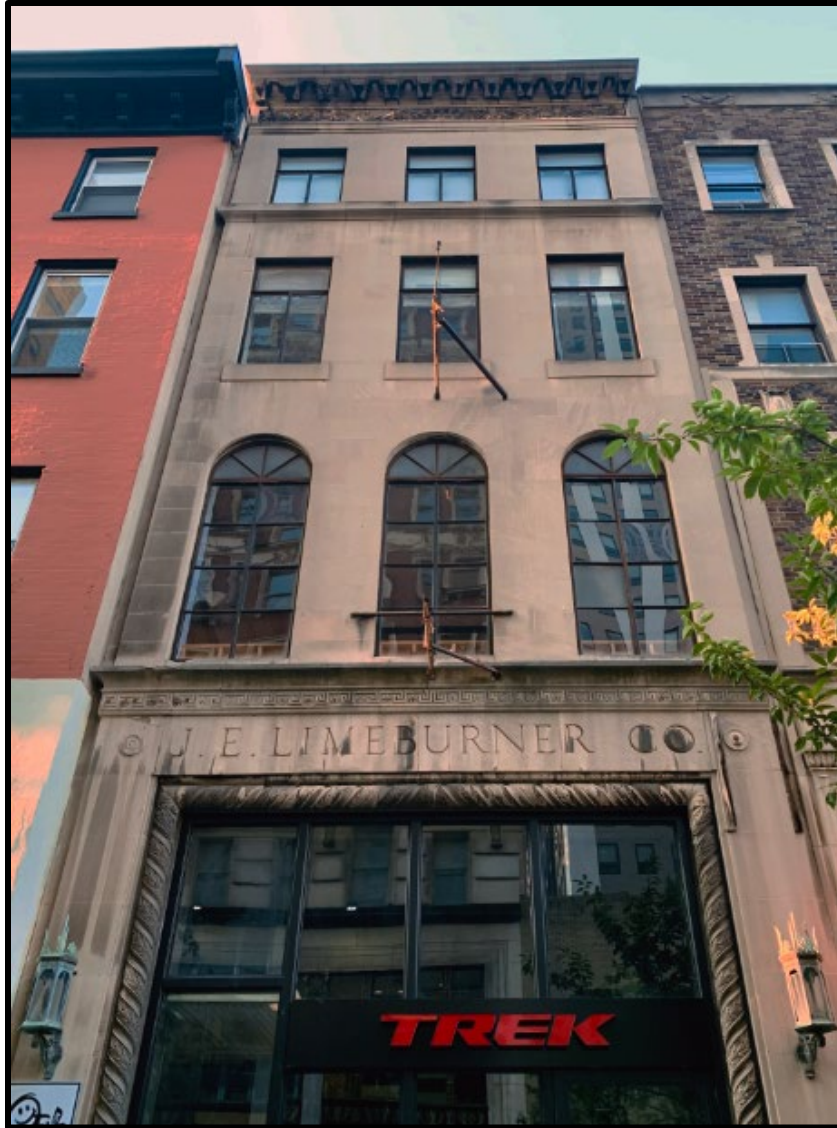
Figure 3. The primary (south) elevation of the J.E.Limeburner Store. Source: Oscar Beisert, 2020.
