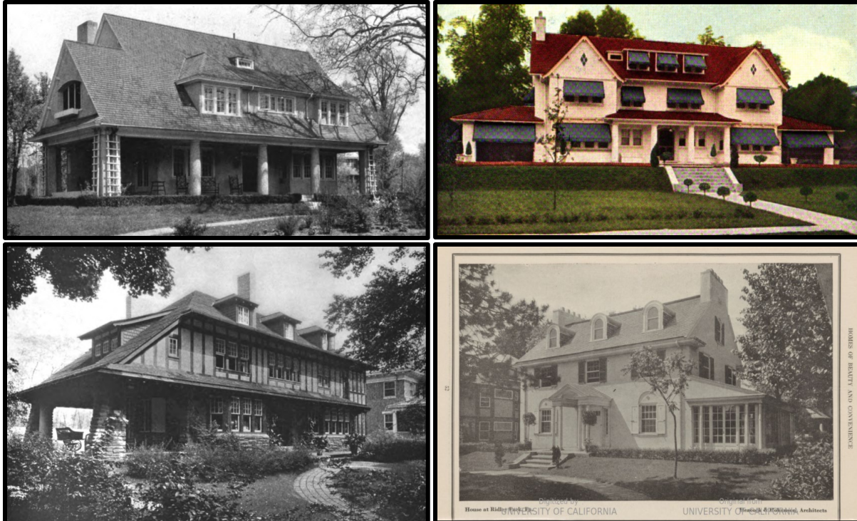
Residential designs by Heacock & Hokanson. Figure 28. Top left: House at Lansdowne, Pa. for Mr. Charles S. Musser. Source: The Western Architect , February 1917, 16. Figure 29. Top right: The W.P. Moore Residence, Elkins Park, Pa., designed by Heacock & Hokanson. Source: The Roof Beautiful: A Simple and Concise Story of the Origin and Use of Roofing Tiles . (Chicago: Ludowici-Celadon, 1921), 9. Figure 30. Bottom left: House for Mr. Joseph L. Heacock, Germantown, PA. Source: The Architectural Review , 1916. Figure 31. Bottom right: House at Ridley Park, designed by Heacock & Hokanson, Architects. Source: Homes of Beauty & Convenience . (New York: Building Age & The Builders' Journal , 1923), 52.
