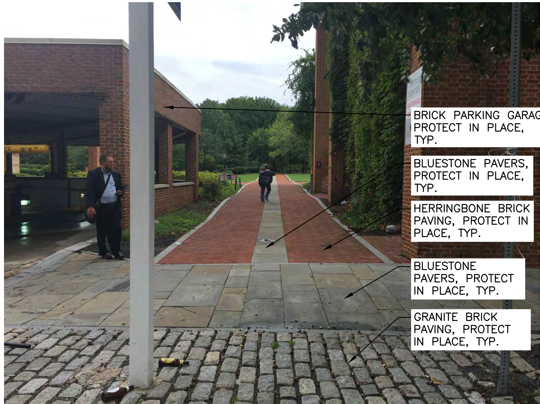
AREA G: EXISTING CONDITIONS
