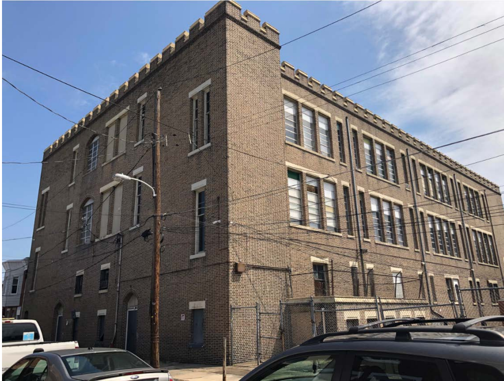
View from Joyce Street of the northwest and southwest elevations.
