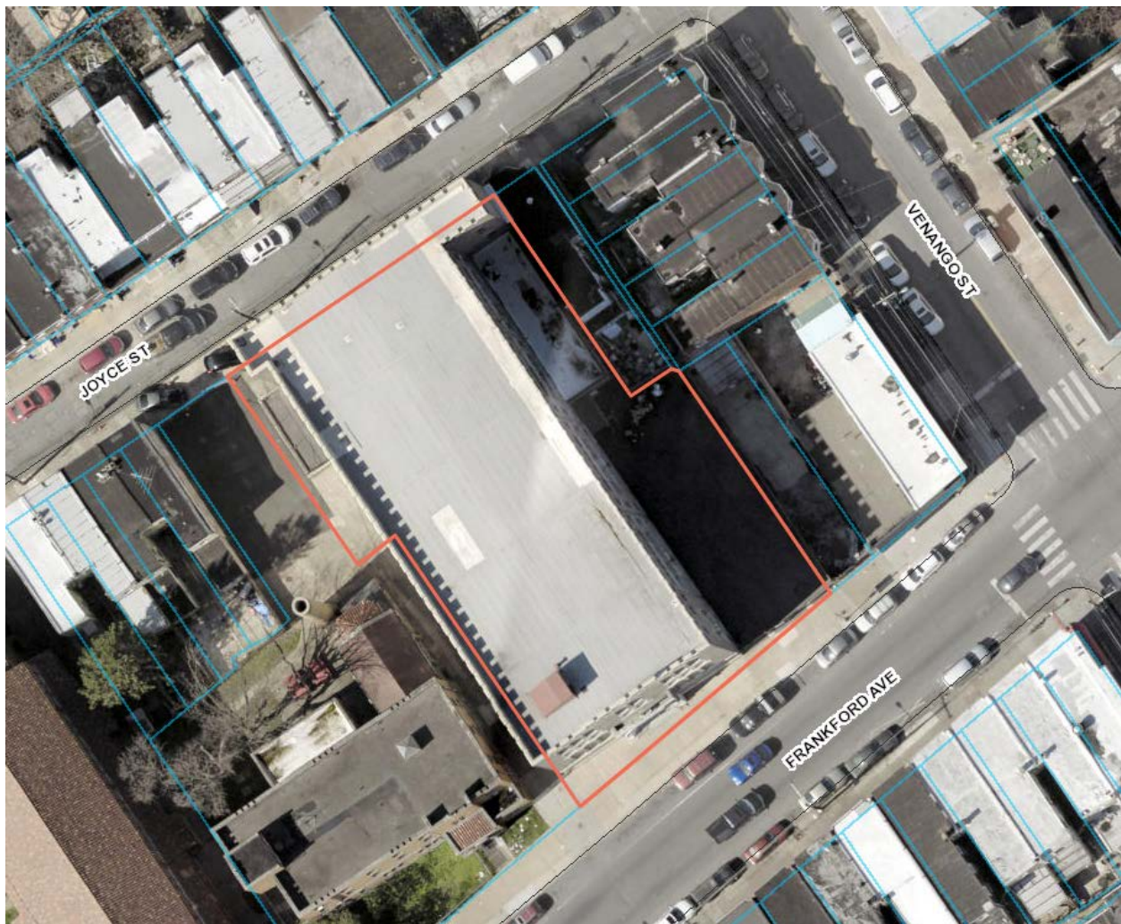
The boundary of the parcel at 3568 Frankford Avenue, shown in orange. The roof of the 1946 St. Joan of Arc Church is visible in the lower lefthand corner of the image.
