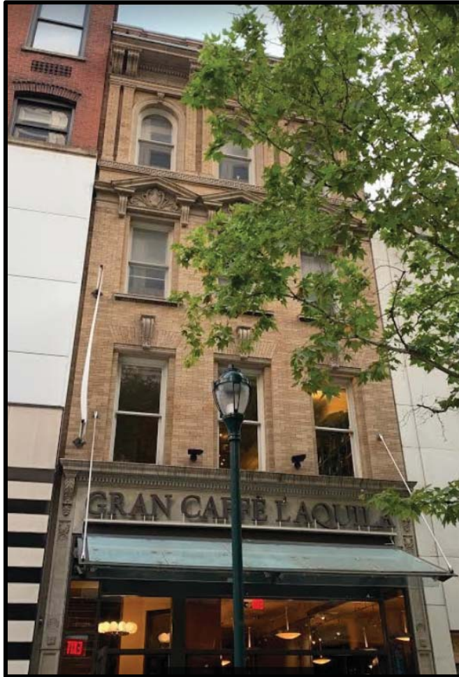
Figure 1. The primary (north) elevation of the Wall & Ochs Building. Source: Oscar Beisert, 2020.
