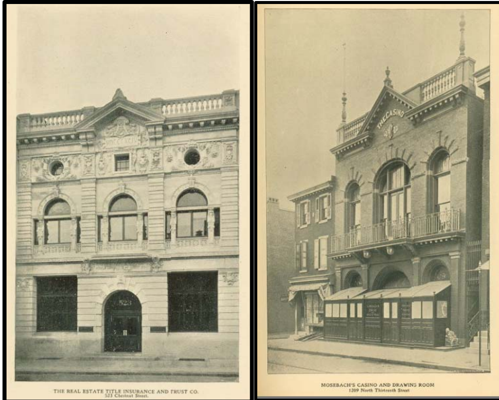
Two variants of the Renaissance Revival style on a small scale in Philadelphia. Figure 52. Left: The Real Estate Title and Trust Co. (Demolished) at 523 Chestnut Street, opposite Independence Hall. Figure 53. Right: Mosebach's Casino and Drawing Room (Demolished) at 1209 North Thirteenth Street.
