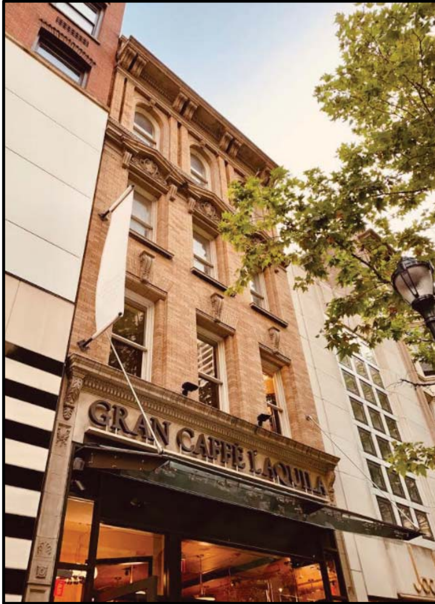
Figure 3. The primary (north) elevation of the Wall & Ochs Building. Source: Oscar Beisert, 2020.
